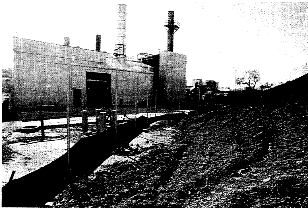
Classified Waste Incinerator Under Construction
