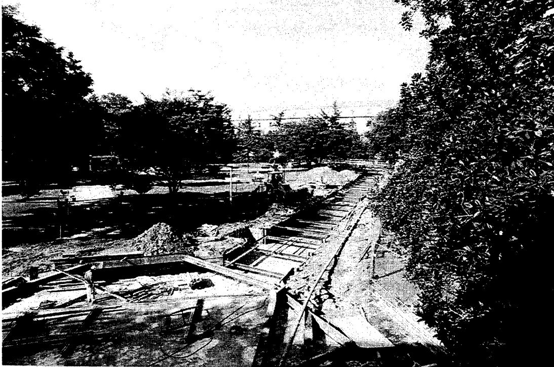
Center Courtyard Utilities Tunnel Under Construction
