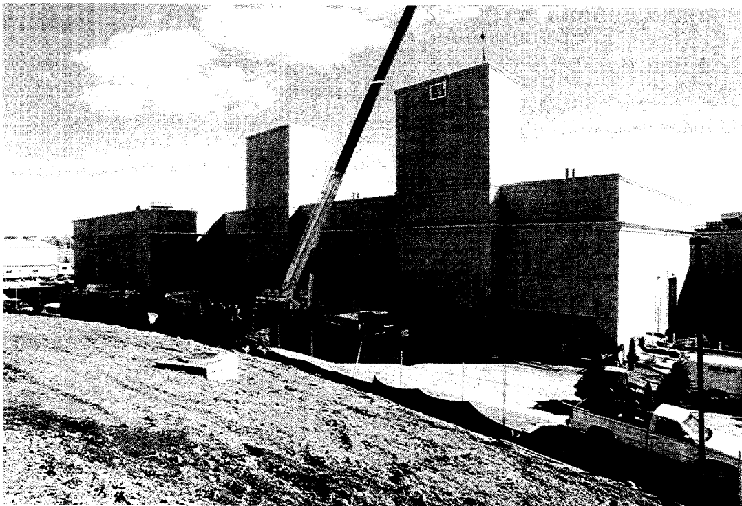
Heating & Refrigeration Plant Under Construction
