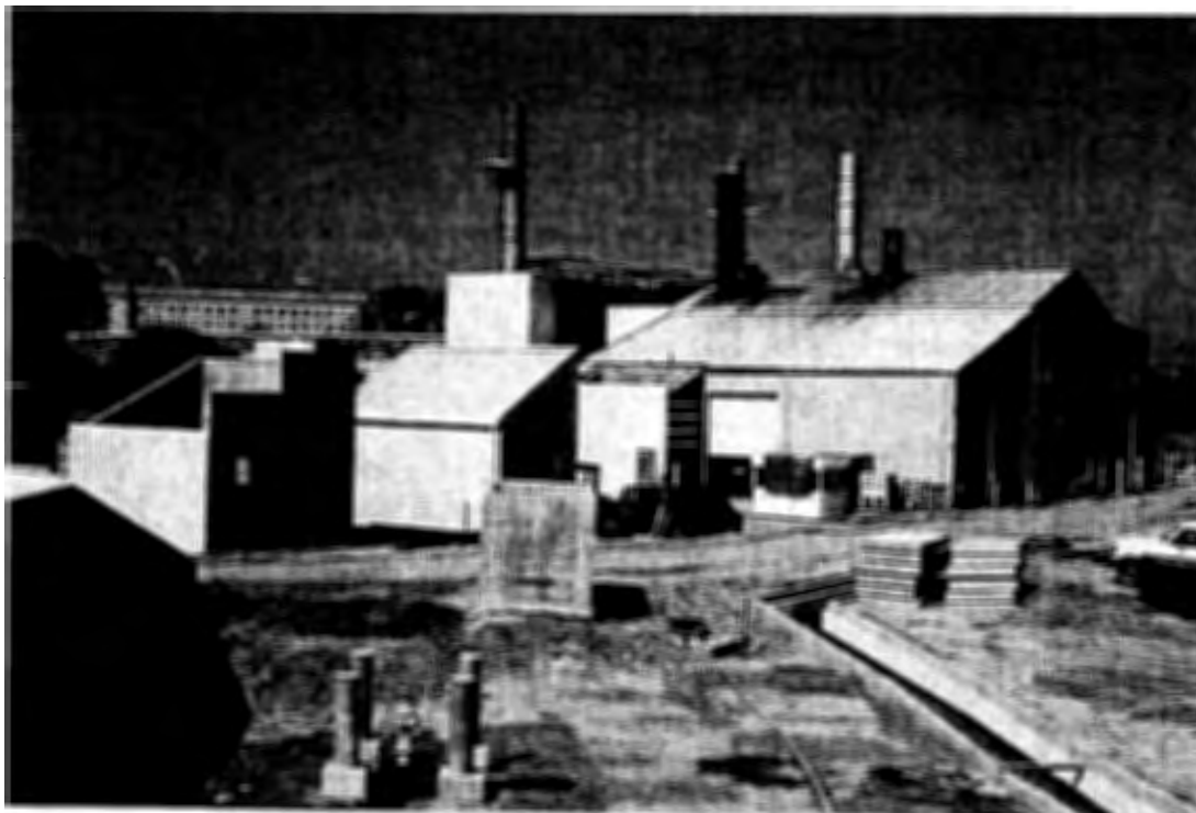
Classified Waste Incinerator Under Construction
