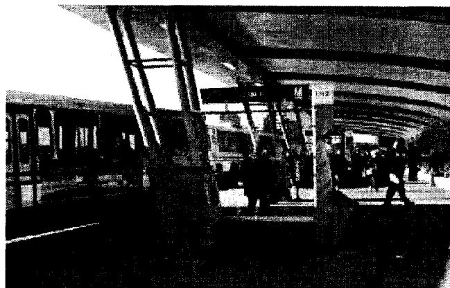
During construction of the new bus facility recycled materials were used. Recycled concrete was used for the base material of all roadways and sidewalks
