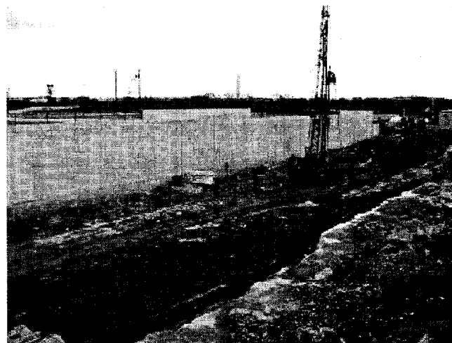
A view of the 100-foot zone from the Pentagon Mall Terrace.
