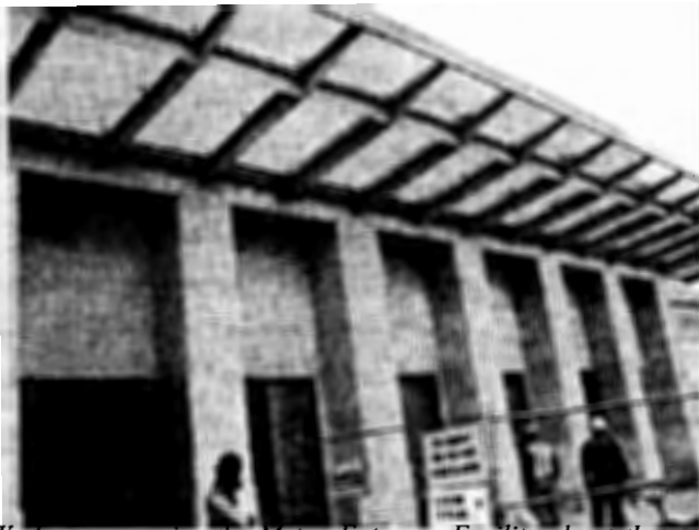
Workers surveying the Metro Entrance Facility about three weeks prior to the Grand Opening.
