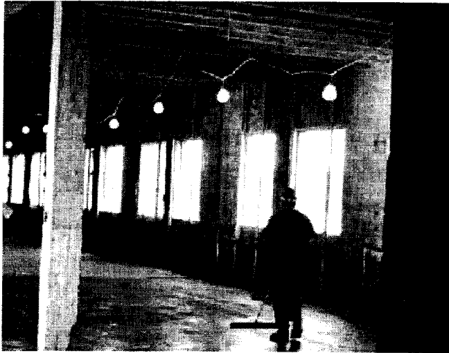
Inside, after demolition and abatement of space is complete.
