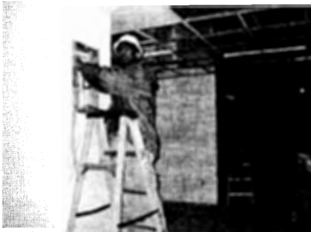
Installing phone lines in Wedge 2
