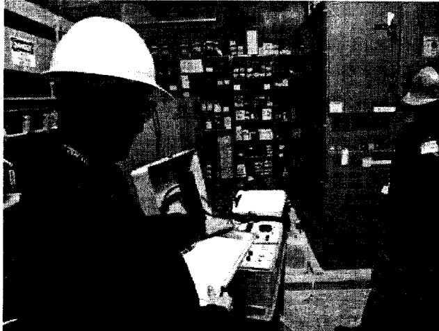
Above, workers testing a Wedge 1 electrical vault. The original vault was destroyed in the September 11 attack. This particular test measured the integrity of the wiring that feeds the vault. Below, Wedge 2 Quality Assurance Inspectors on a weekly project walk-thru.
