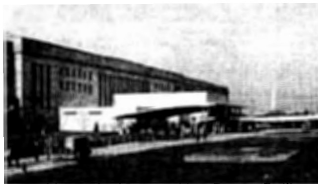
A view of the completed Pentagon Metro Entrance Facility (MEF). The MEF was completed on schedule, despite construction delays caused by the 9/11 terrorist attack. The entrance facility and bus loop are designed to adequately handle the 34,000 daily commuters who take the bus or Metro Rail to the Pentagon.
