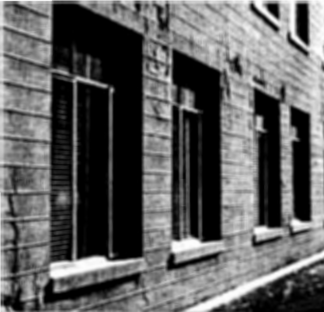
In addition to improving the appearance of the building facade, the Pentagon Renovation Program is installing new, energy efficient windows. The old windows contribute to a 30% energy loss in the unrenovated parts of the building.
