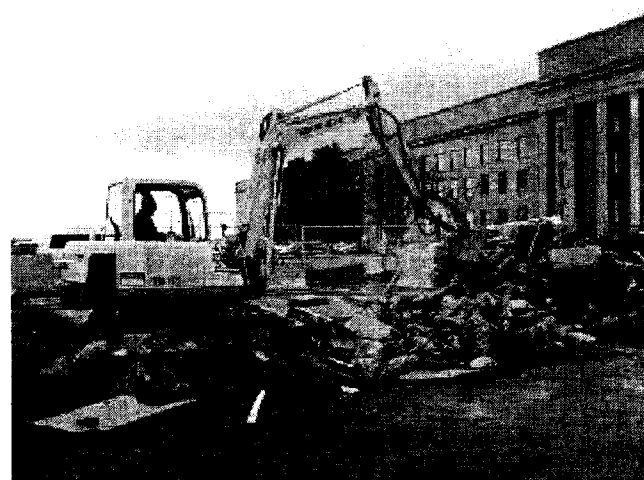
Workers begin the waterproofing process for the PAC on the Mall Terrace parking lot.
