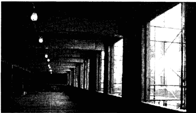
Wedge 2, immediately after demolition, ready for Core & Shell Construction.
