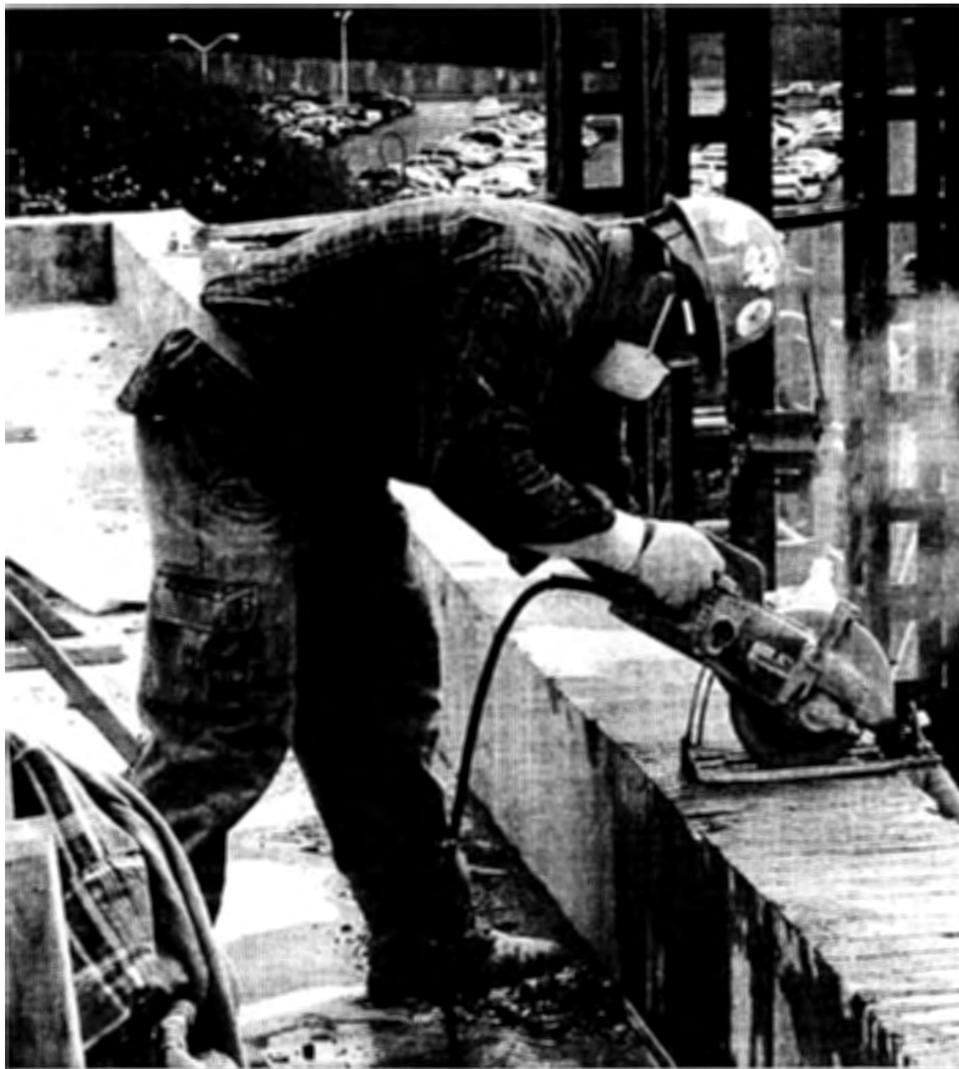
A Phoenix Project worker cutting limestone for the building facade
