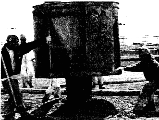
April 5, 2002: The final concrete pour. The structure of the Phoenix Project reaches substantial completion just 7 months after the terrorist attack.
