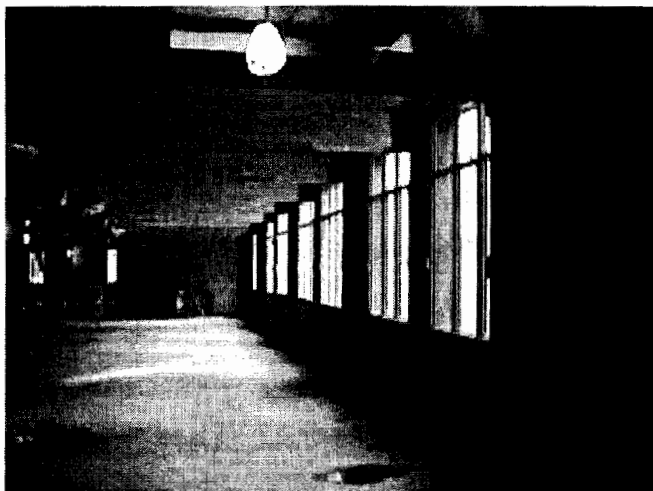
These photos show Wedge 2 areas on the fourth floor, where demolition has been completed and core and shell work has begun. In the top photo, new windows have been installed. Below, a view of some initial ductwork.
