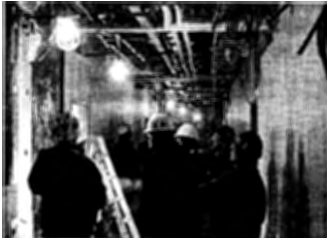
Above, workers testing a Wedge 1 electrical vault. The original vault was destroyed in the September 11 attack. This particular test measured the integrity of the wiring that feeds the vault. Below, Wedge 2 Quality Assurance Inspectors on a weekly project walk-thru.
