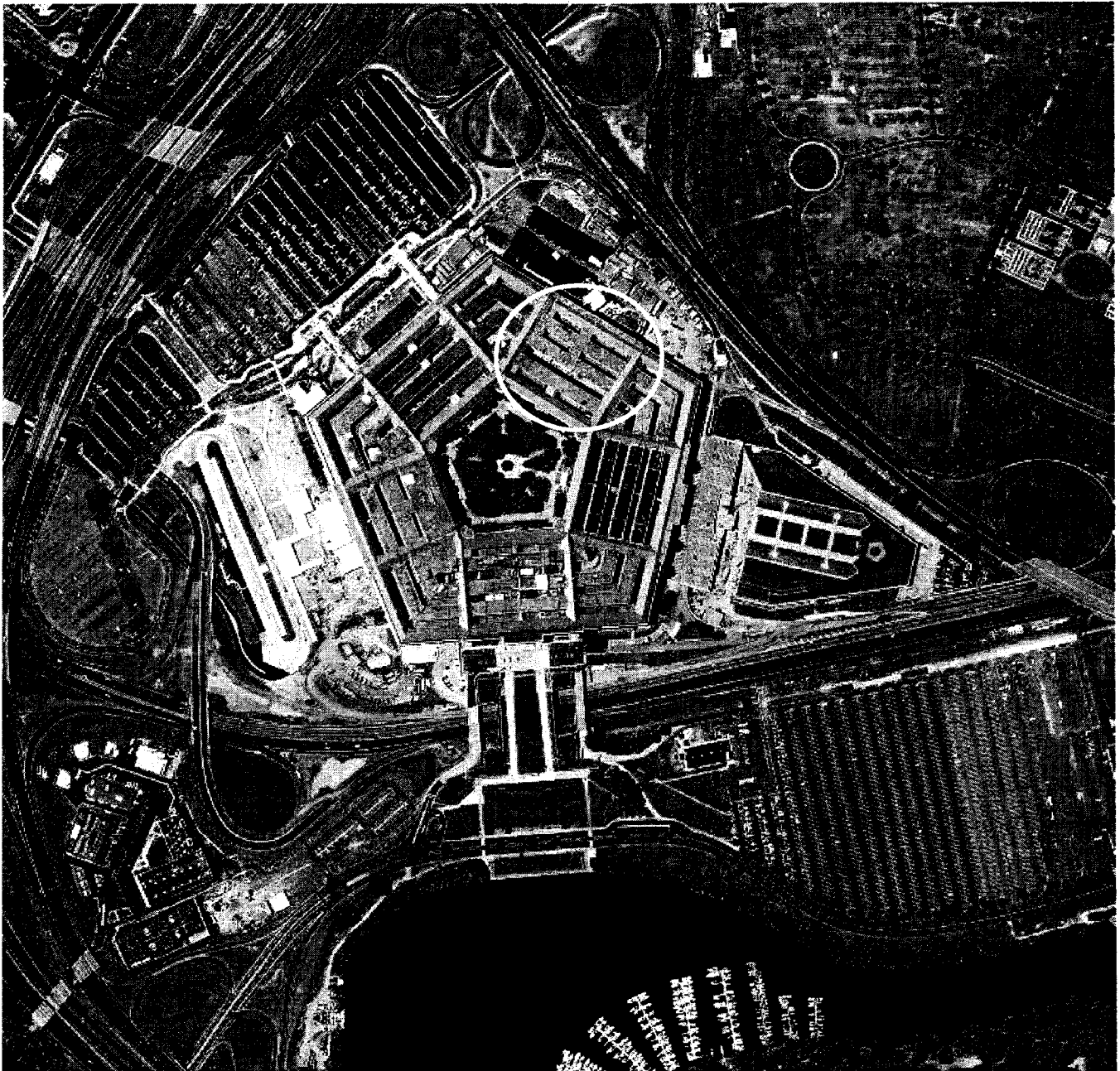
An aerial view of the Pentagon Reservation, taken on September 7, 2002, less than one full year after the terrorist attack on September 11, 2001. The photo illustrates the completed structure of the Phoenix Project (circled).
