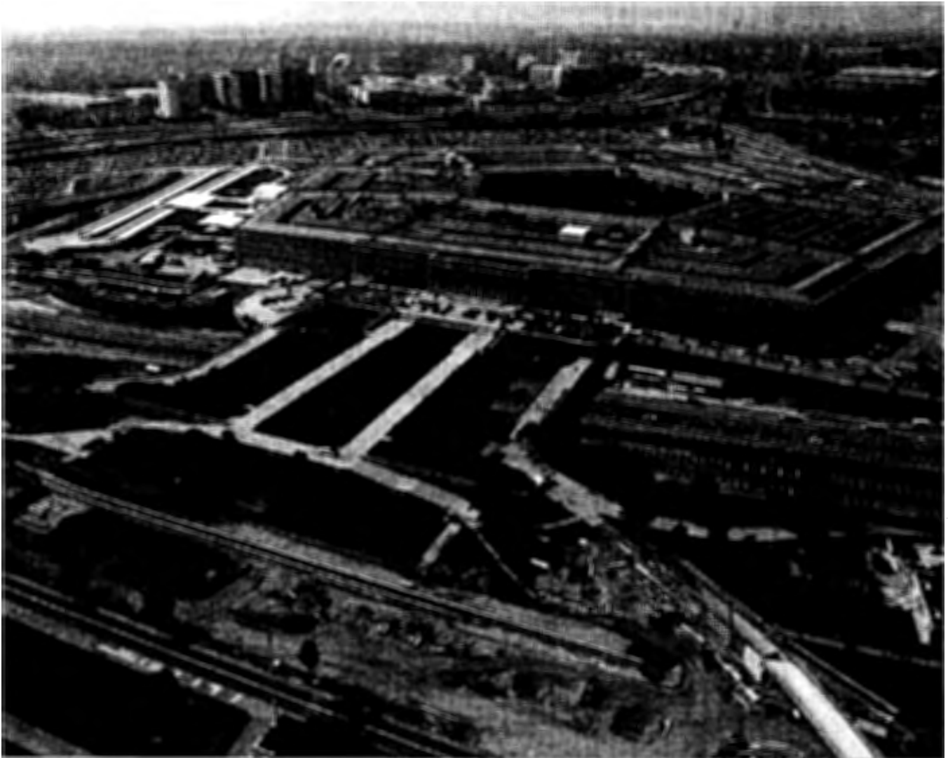
This September 2003 picture provides a good aerial view of the progress made by the Roads, Grounds and Security Team's work to relocate Highway 110 away from its original location near the Pentagon.
