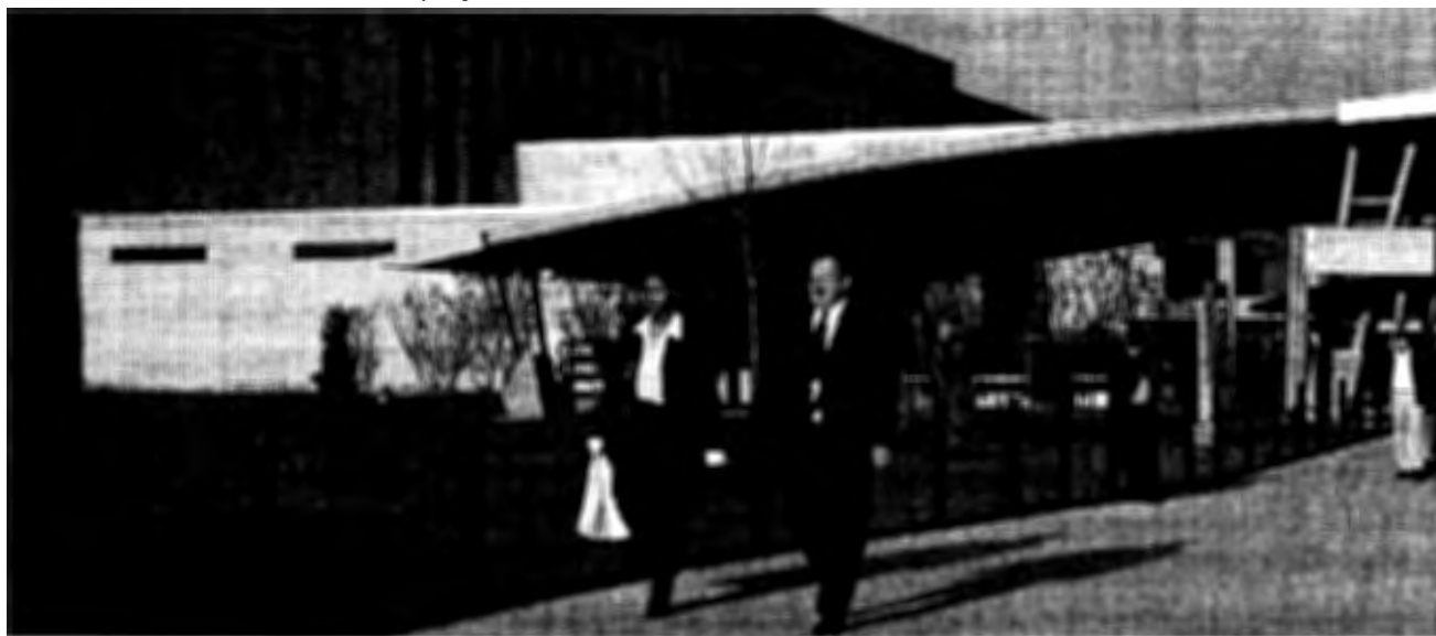
A view of the Pentagon from the Metro Entrance Facility, which was recently awarded LEED TM Certification. The MEF was the first federal building in the National Capital Region to achieve this certification.
