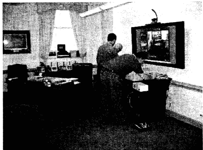
Technicians installing equipment in one of the Army Senior Staff offices.
