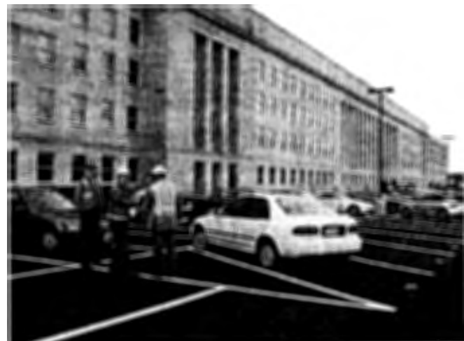
Construction is complete on a new Executive Parking Lot outside the Corridor 5 Entrance.
