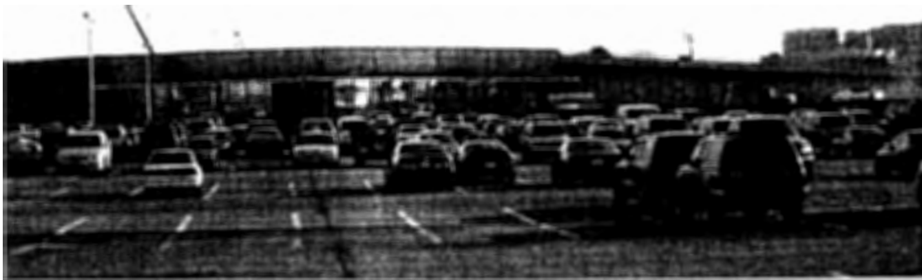
This photo shows the North Parking connector bridge that will span the relocated Highway 110. The Pentagon Secure Bypass (PSB) routes traffic on Highway 110 away from the building, through what is now the Pentagon North Parking Lot. When the project is finished, it will enable DoD to lift the current truck restrictions on Highway 110.
