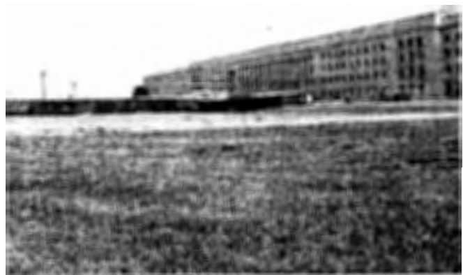
The two acre site of the Pentagon Memorial Project has been cleared out for construction.
