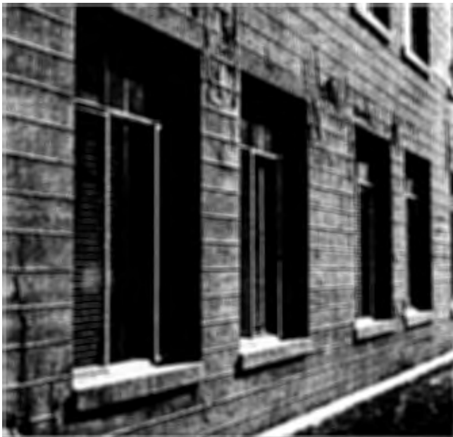
In addition to improving the appearance of the building facade, the Pentagon Renovation Program is installing new, energy efficient windows. The old windows contribute to a 30% energy loss in the yet to be renovated parts of the building.
