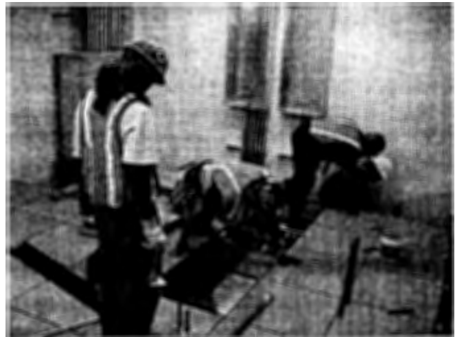
Workers installing a raised floor in the Basement Area.
