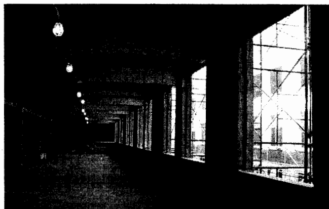
Complete, slab-to-slab demolition strips the space down to the concrete structure.
