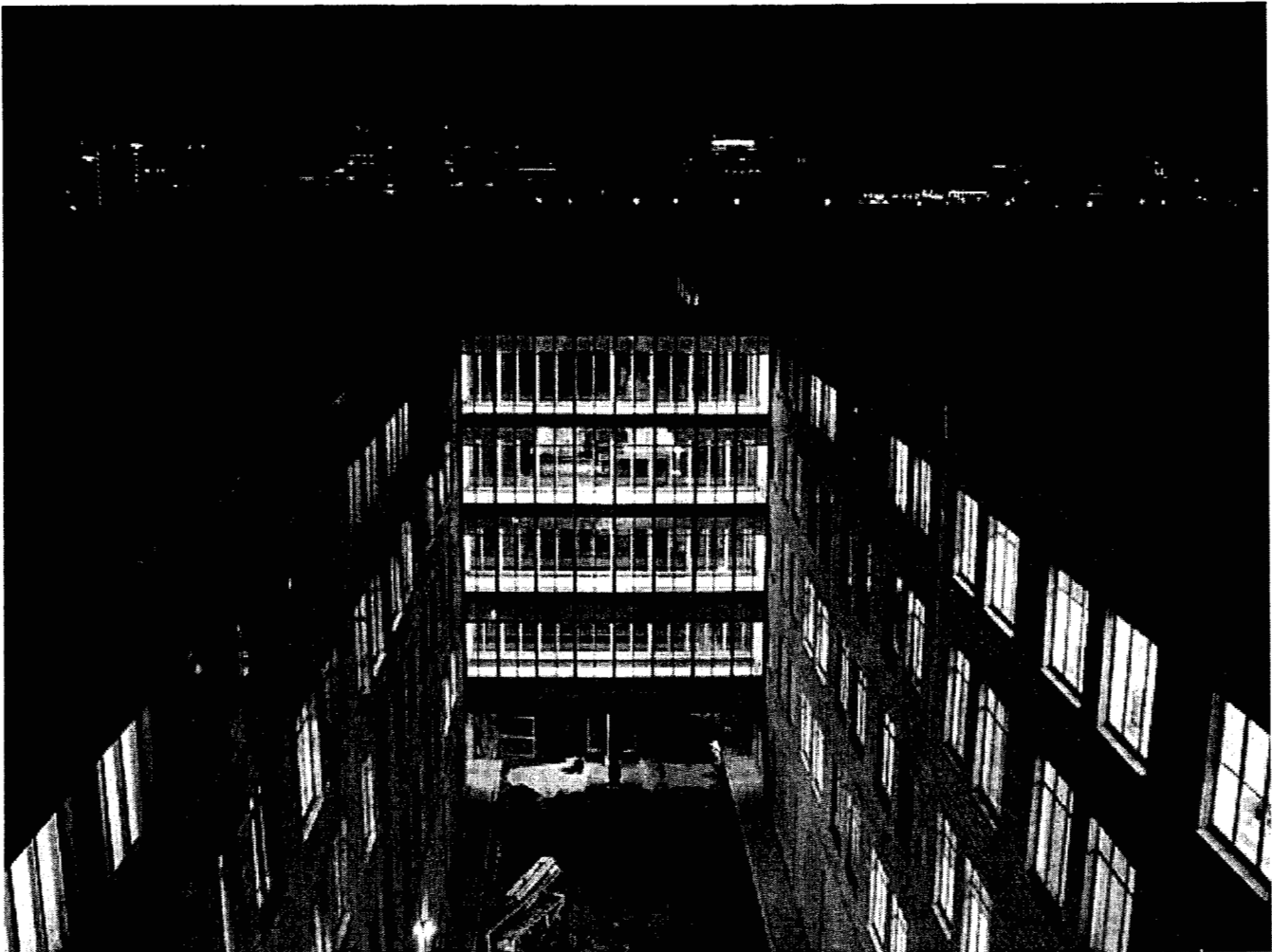
A nighttime view of A-E Drive. The renovation of Wedges 2-5 includes the addition of "half corridors" which will flow continuously from the A-ring to the E-ring. Glass bridges, like the one shown here for Corridor 4.5, will span the light wells for maximum building access and egress. These walkways will also increase use of natural light.
