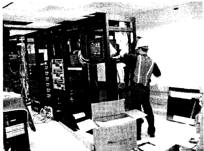
Workers installing equipment in the editing suite of the new OSD Public Affairs area.
