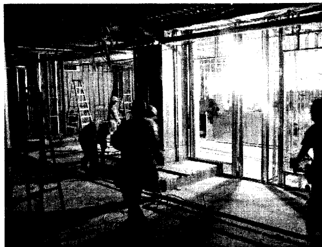
Wedge 2 core and shell construction.
