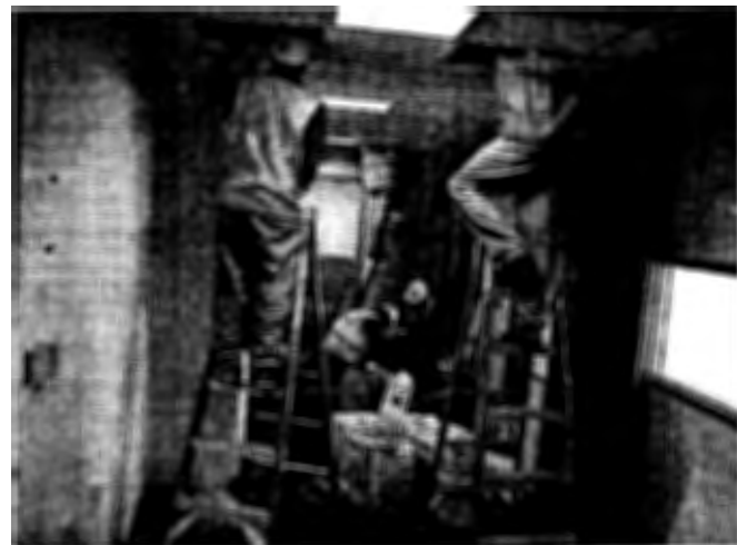
Electricians pulling wiring in a nearly completed Wedge 2 space.
