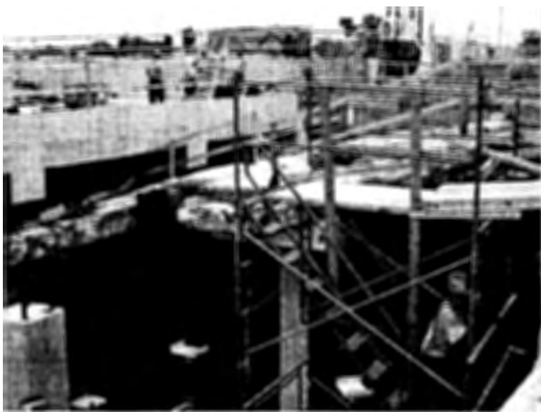
Workers complete the concrete exterior structure of the PAC.
