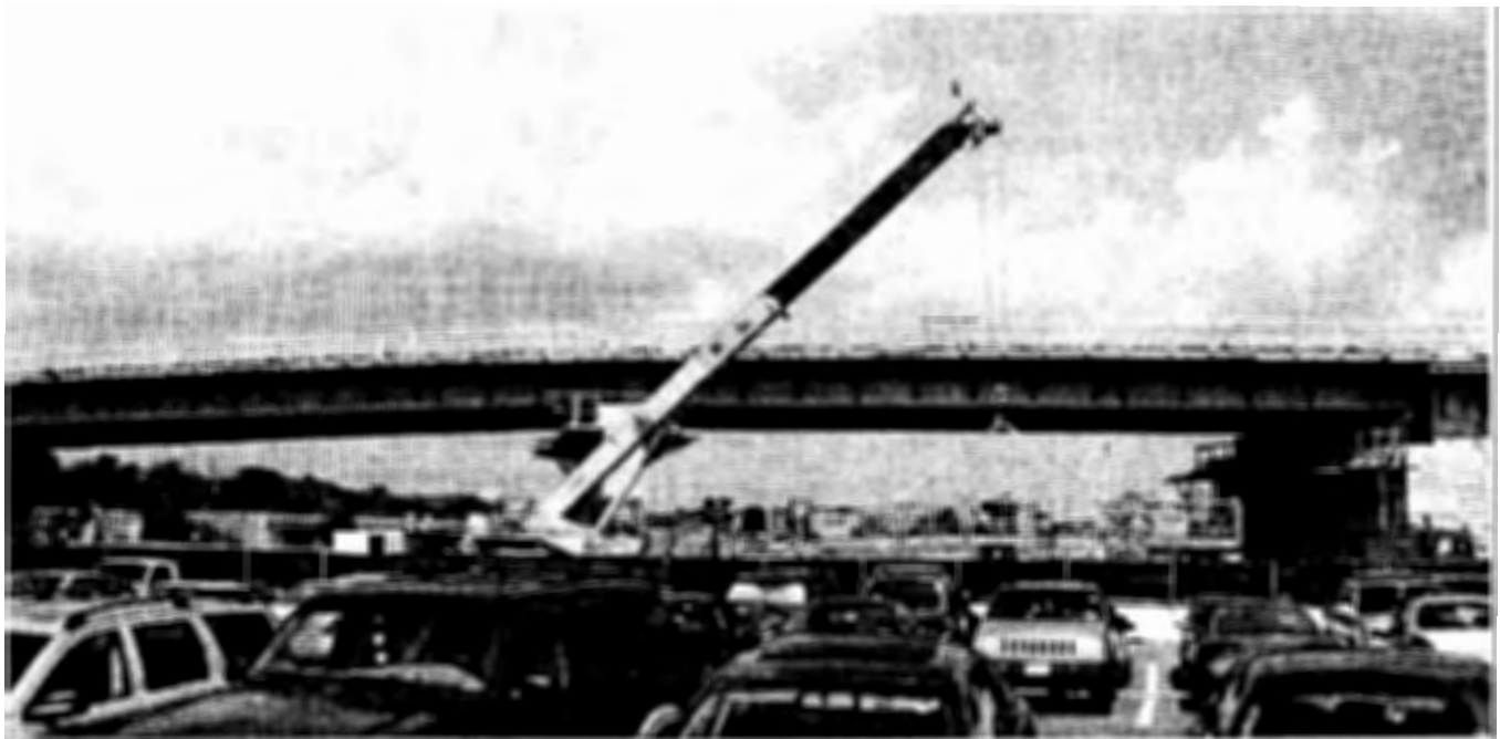
The new vehicle access bridge, which spans Highway 110 and provides access to new parking areas in North Parking.
