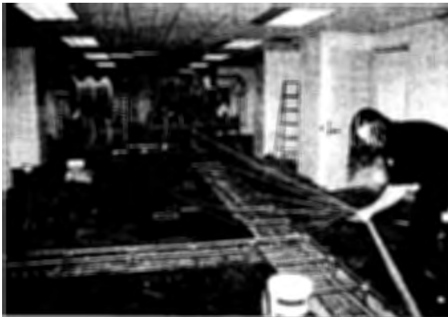
A technician pulls new fiber optic lines from large spools.
