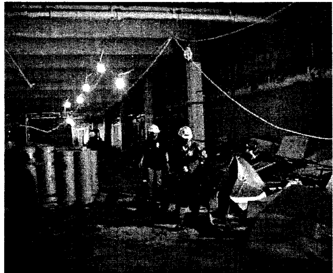
View inside Phase 1 showing mechanical demolition and debris removal.
