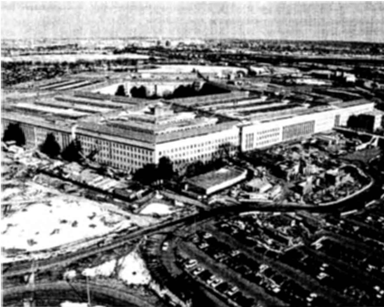
Aerial view of the Pentagon as it appeared in February 2000. Construction of the second pedestrian bridge at Corridor 3 continues along the South Terrace (right). Trailers dedicated to the Wedge 1 team can be seen to the left of the bridge construction area (center of photo). The Wedge 1 construction staging area can be seen on the Heliport side (left).
