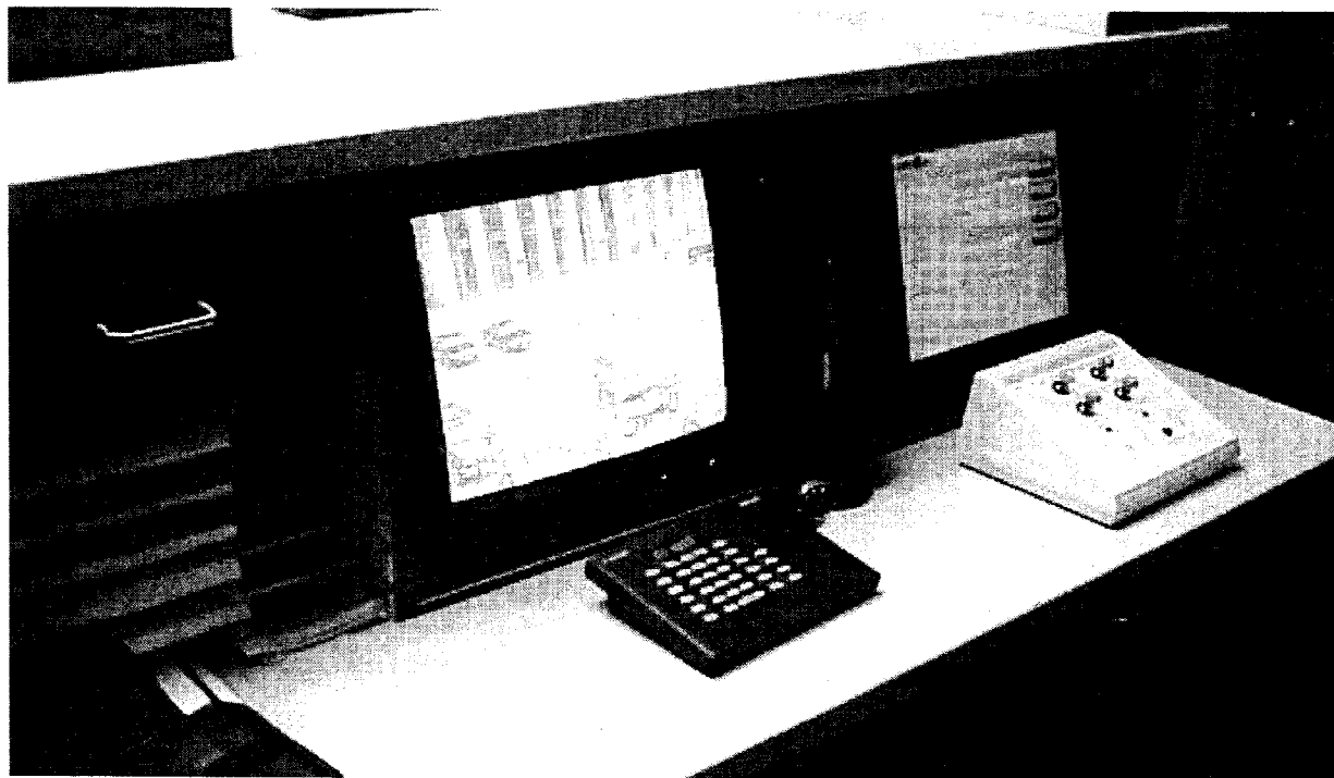
A state-of-the-art security station with CCTV, Video Image Recognition, Communication, and Bullet Resistance Protection capabilities.
