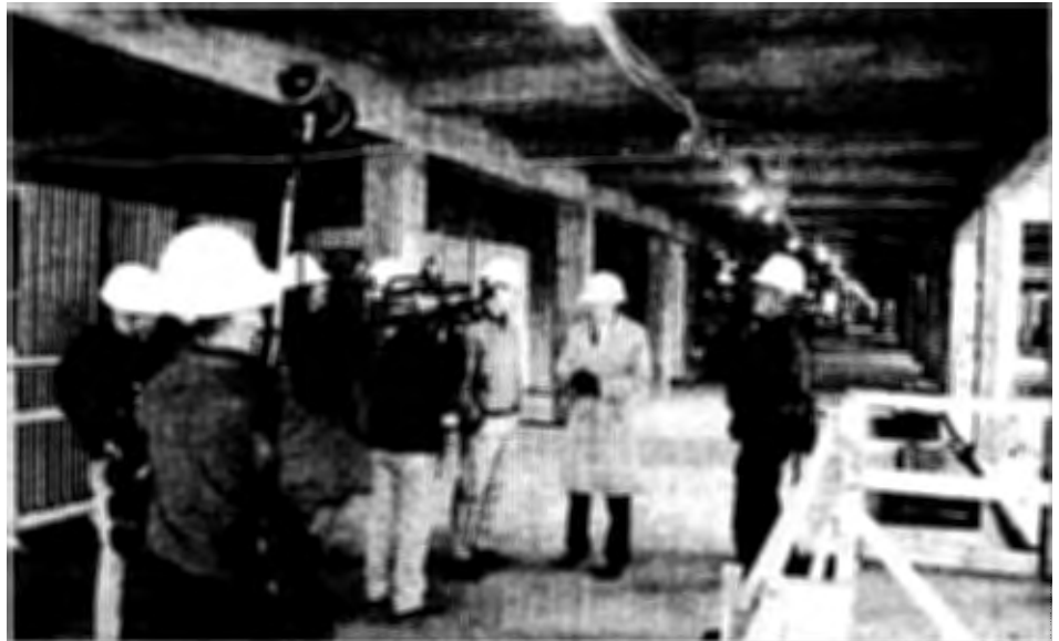
CBS News reporter, David Martin (center, facing right) interviews the Pentagon Renovation program manager inside Wedge 1. The interview will be used in a 60 Minutes II segment about the project expected to air in the spring of 2000.
