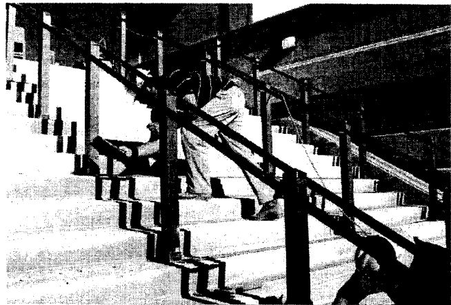
Finishing work on new South Terrace bridge steps
