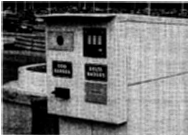
Card reader stanchion with CCTV, intercom, and multi-badge capabilities.
