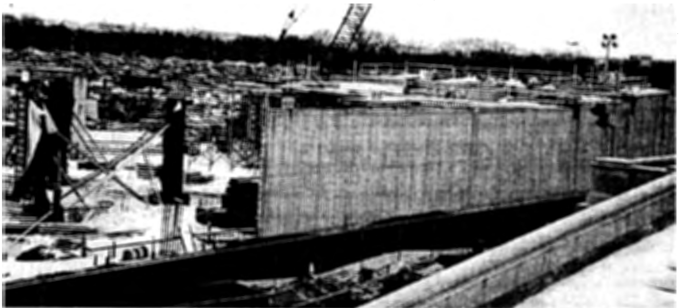
Heavily reinforced concrete walls continue to rise on the site of the Pentagon's new Remote Delivery Facility.
