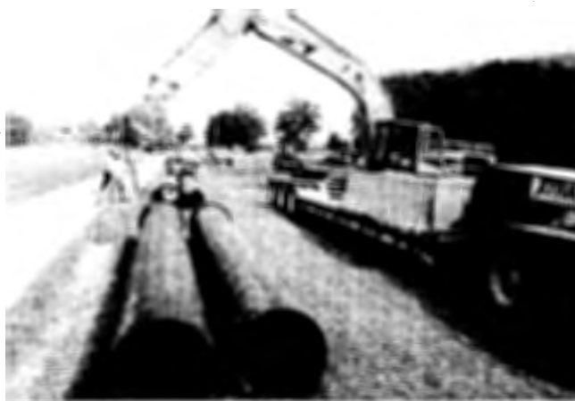
Work on new chilled water lines near the Heliport
