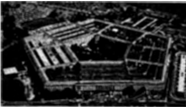
Aerial view of the Pentagon. Wedges 1-5 encompass 5,000,000 square feet of building space above ground.
