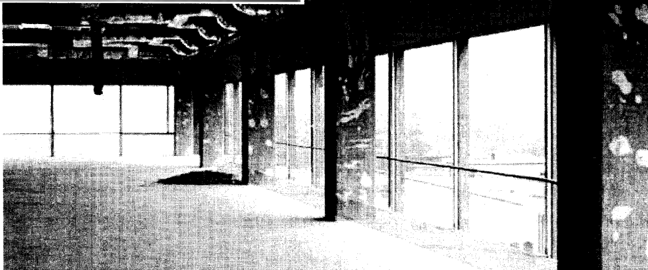
Above: A swing space area ready for new stud walls that will define the tenant space. Inset: Systems furniture in place.
