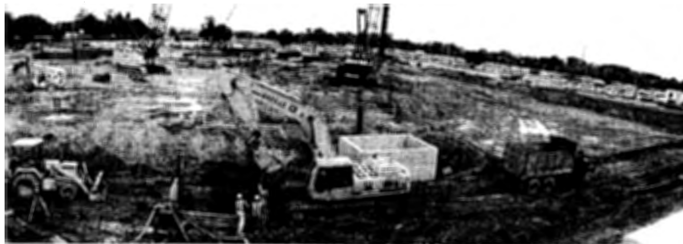
June 1999, a panoramic view of the site work for the new Remote Delivery Facility.
