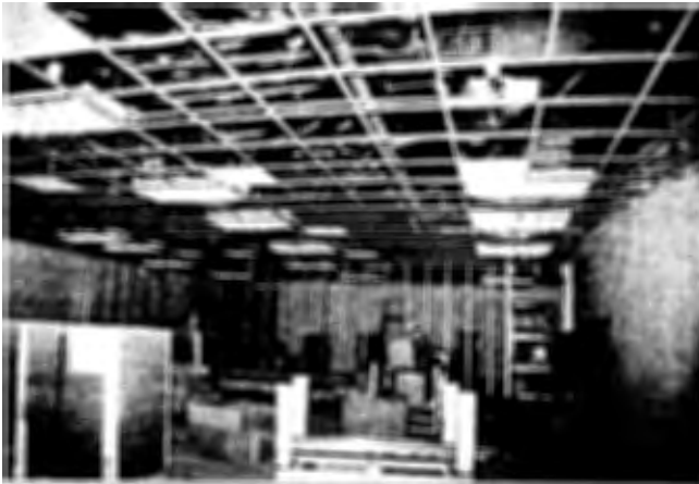
The ceiling grid is installed in the Segment 2A2 basement area. The curved wall at right is the foundation for the roadway above.
