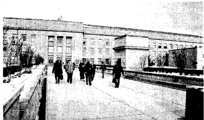
Employees use the new pedestrian bridge at Corridor 2 to safely enter the Pentagon from South Parking.
