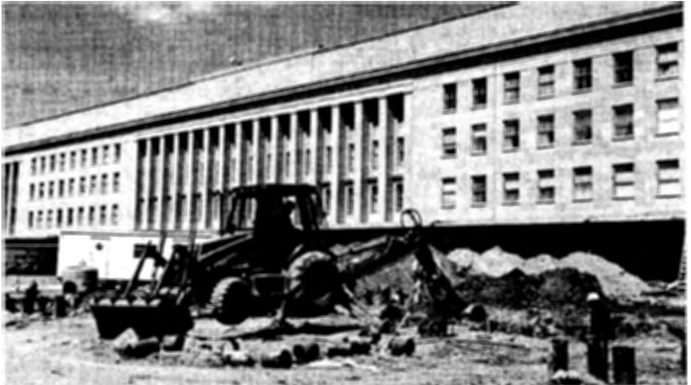
Construction along the Pentagon's South Terrace
