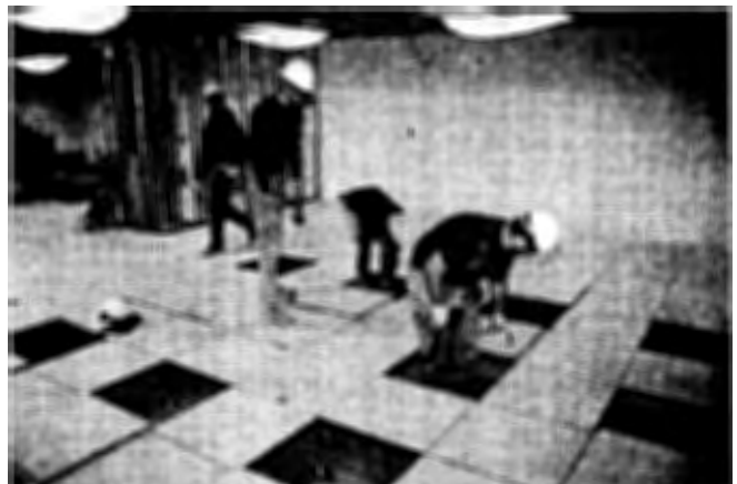
A crew installs the raised floor that will support a new technical facility in the basement.
