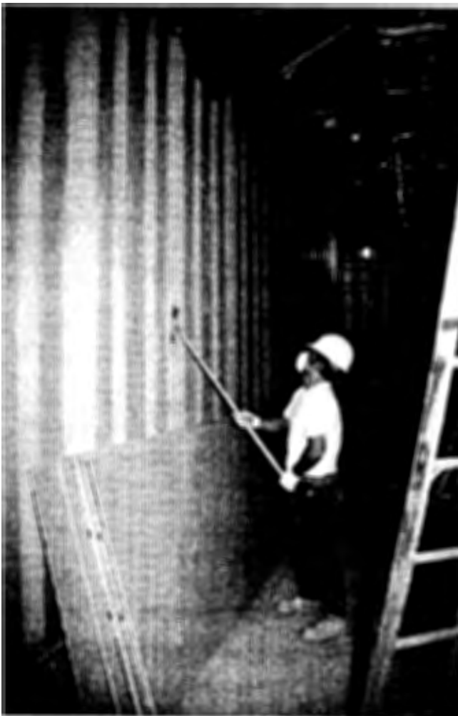
Worker sands the sheetrock to prepare the surface for painting.
