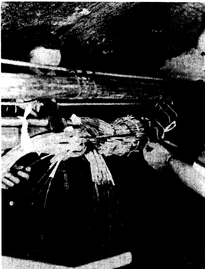
Technicians install original telephone wiring in the Pentagon. Much of it still exists as new systems were laid on top of old. Seldom are changes reflected on existing building drawings.
