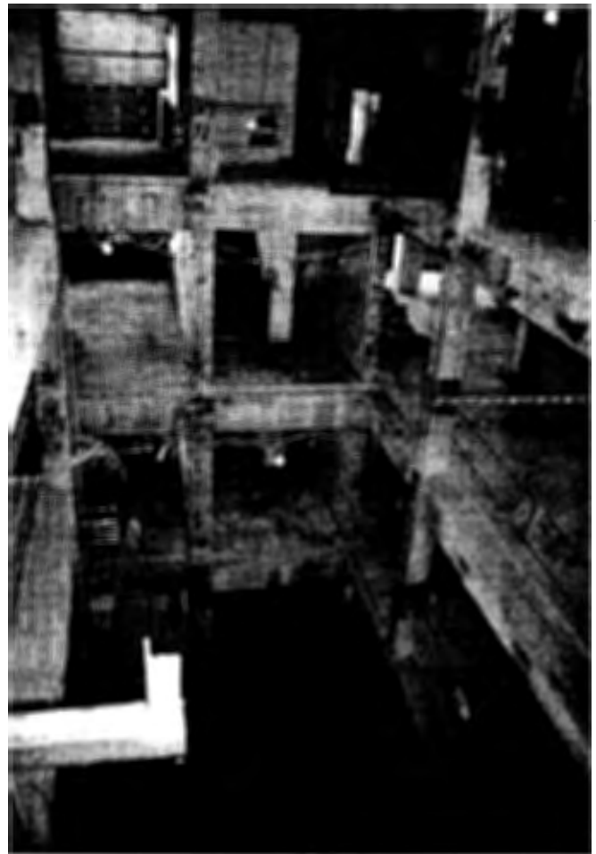
A view inside Wedge 1 where floor slabs have been removed to clear the way for new elevators. Eventually, each wedge will be gutted and cleared down to the bare column structure seen here.
