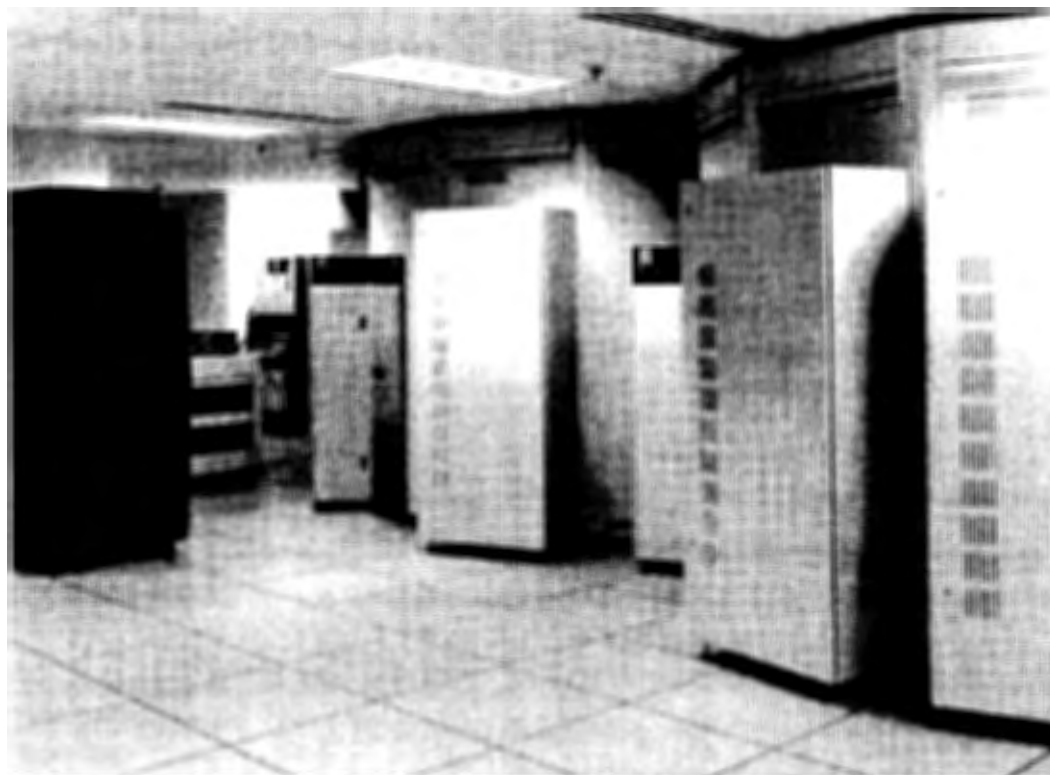
Inside a new data tape storage facility.
