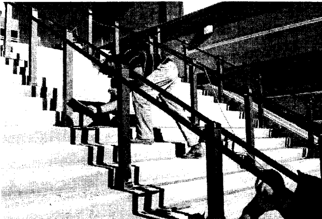
Workers install traction plates on the steps of the pedestrian bridge at Corridor 2.
