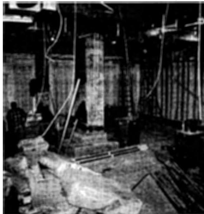
New electrical lines and ductwork is being installed in a portion of the Pentagon basement known as "2A2." Renovation of 2A2 is now complete and the space is fully occupied.
