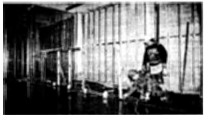
Tenant space is defined as workers in Wedge 1 construct new stud walls.
