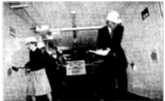
The public affairs program often involves coordination of groundbreaking or ribbon-cutting ceremonies. Above, senior Pentagon officials take part in a ceremonial “wall-bashing” ceremony to mark the beginning of Wedge 1 demolition.
