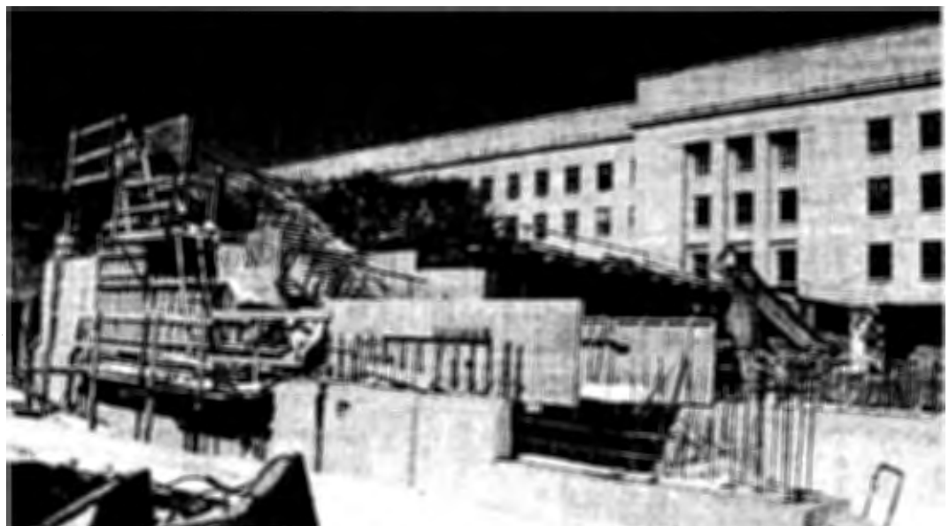
Workers construct the formwork that will give shape to the outer staircases of the Corridor 3 pedestrian bridge.
