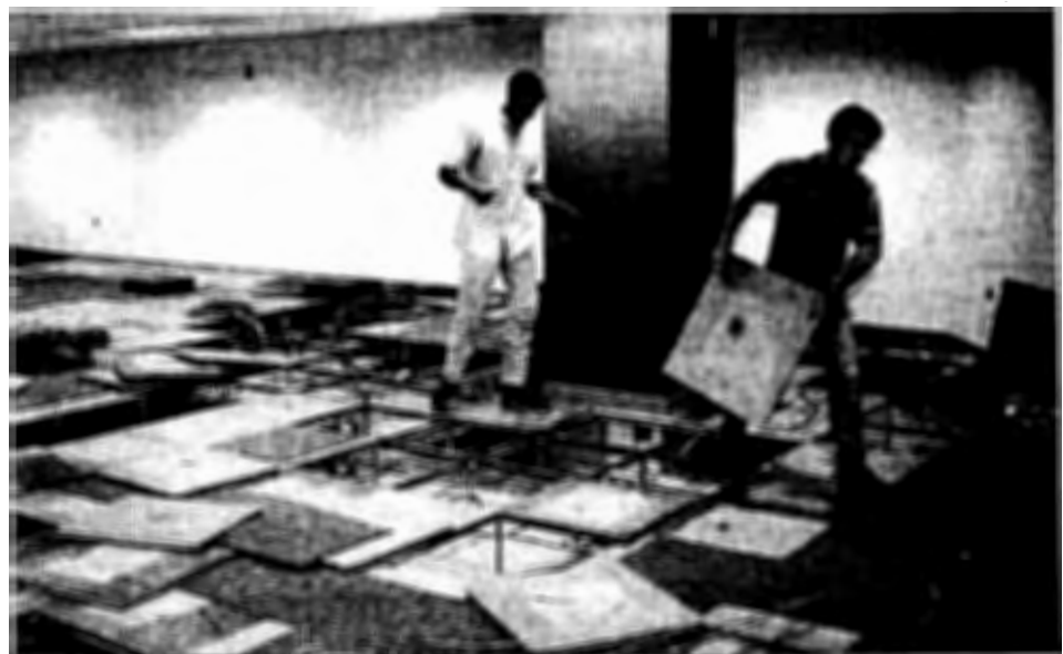
An information management and telecommunications worker removes a floor panel to run new fiber optic lines. The raised floor configuration facilitates changes to office space even after furniture is in place.
