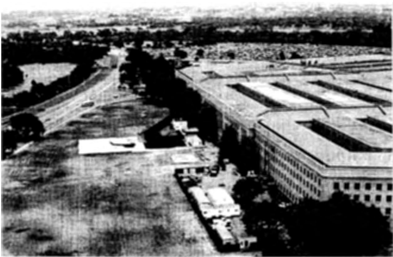
Aerial view looking north at the Pentagon Heliport Fire Station and Control Tower. Renovations are needed to meet the current needs of both facilities.
