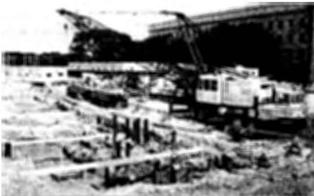
Pile work began for the South Terrace bridge at Corridor 3. The bridge will open concurrently with Wedge 1.
