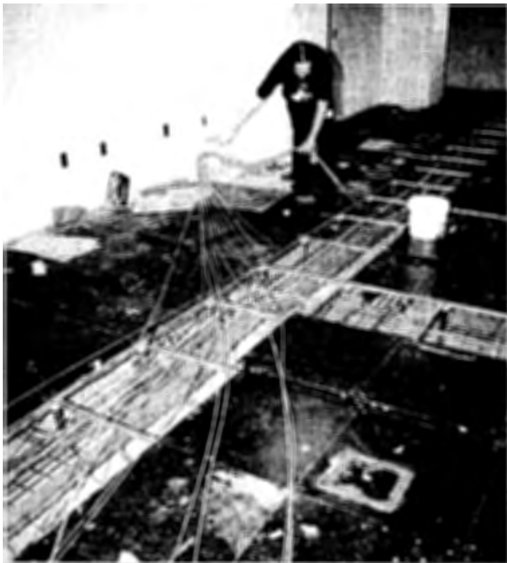
New fiber optic cabling is installed below the raised floor grid.
