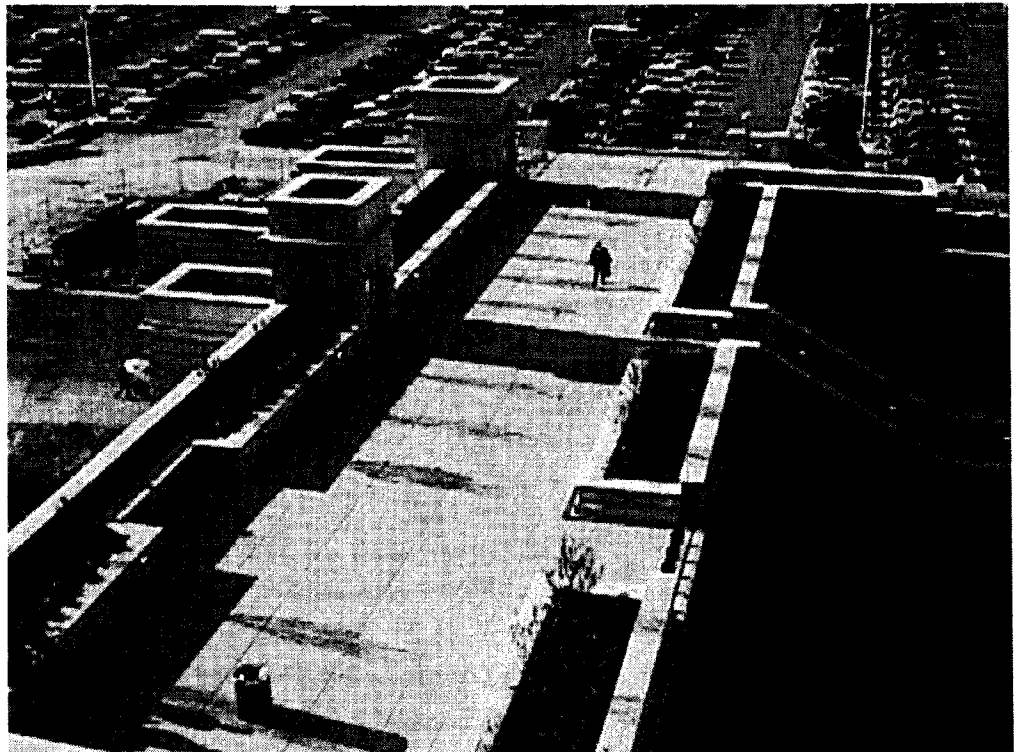
A view of the pedestrian bridge at Corridor 2 from the Pentagon. South Parking can be seen at the top of the photo.
