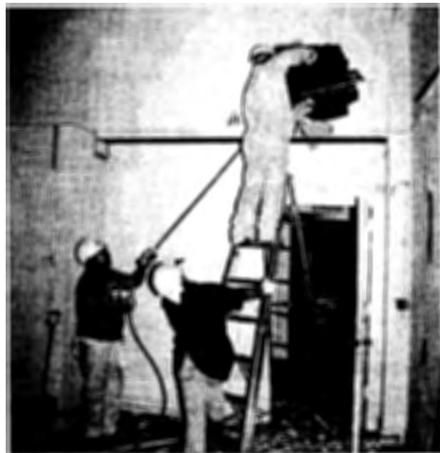
After all utilities have been rerouted, workers begin removal of old wires and conduits hidden within the walls of Wedge 1.
