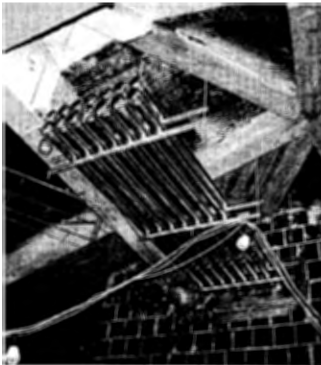
New telecommunication conduits in Wedge 1. Old conduits have been terminated and rerouted.
