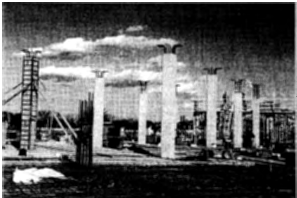
Heavily reinforced columns rise on the Remote Delivery Facility site.
