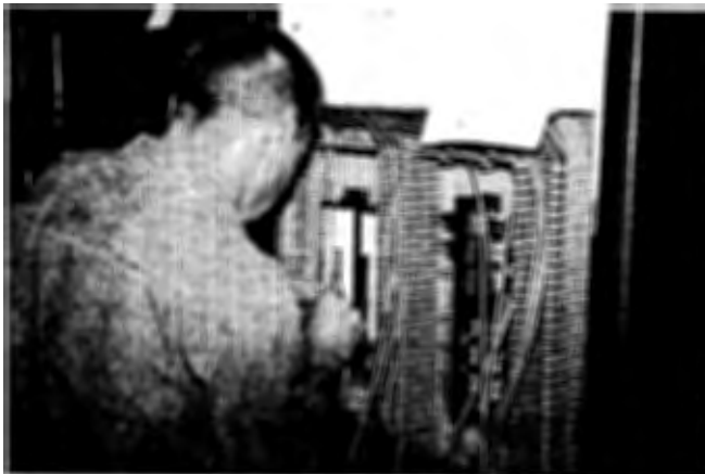
An IT specialist connect data lines to a new spine-wall panel.
