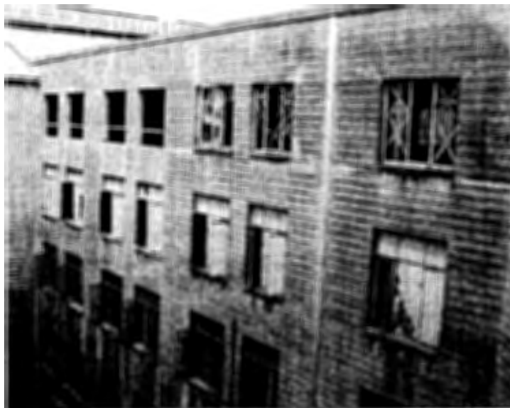
All 7,748 Pentagon windows need replacement. New double-paned thermal insulated units will greatly improve the energy efficiency of the building and enhance security.
