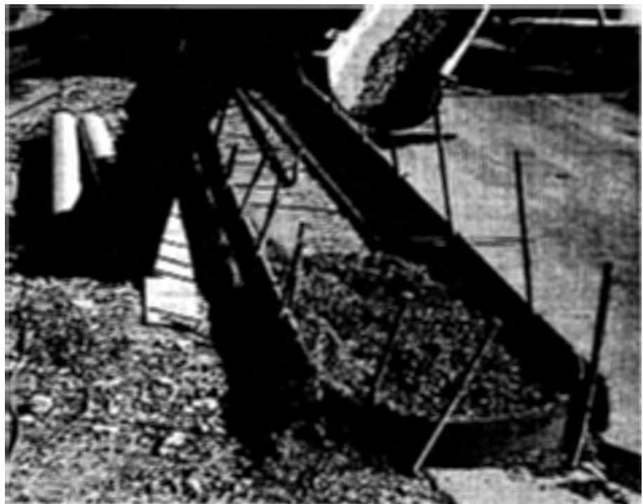
Island at River Terrace for gate arm and card reader has been formed. Concrete placement is underway. Crash bollards to the left of the formwork were installed during the pour.
