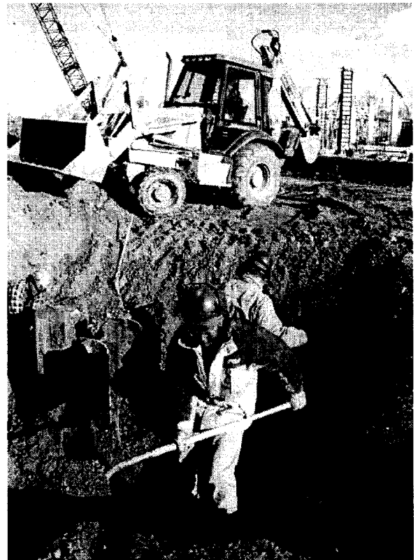
Workers excavate soil near new pilings.
