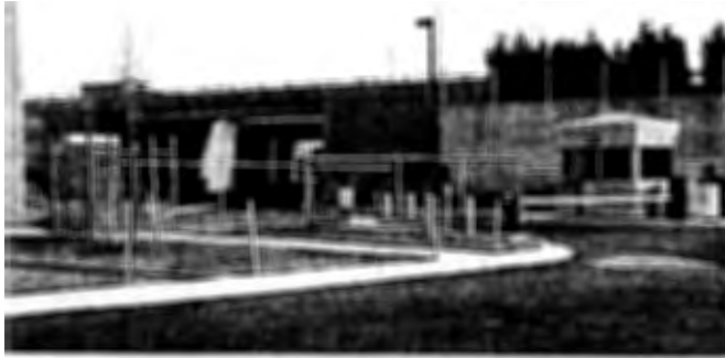
Perimeter access at Utility Plant with crash-rated barrier protection.
