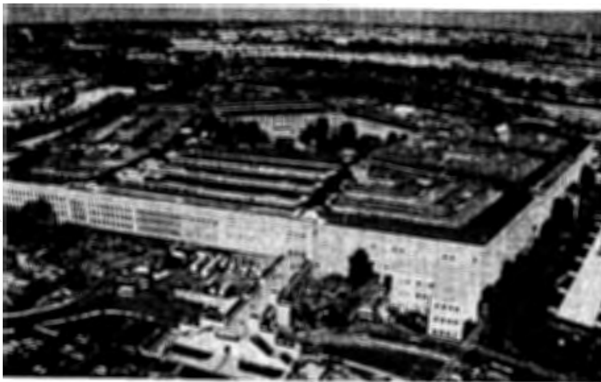
Aerial view of the Pentagon's South Terrace in February 2000. Renovation activities now can be seen in or around all five sides of the building.
