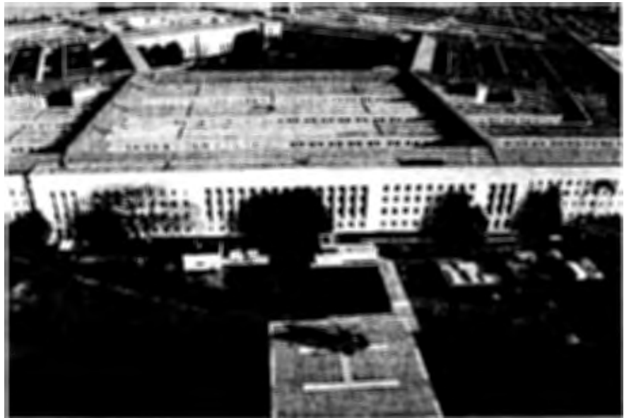
Aerial view of the Pentagon Heliport Fire Station and Control Tower.
