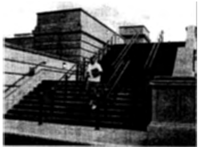
Pentagon employees take advantage of the new pedestrian bridge at Corridor 2 to bypass three lanes of traffic on Rotary Road, which lies between the Pentagon and South Parking.
