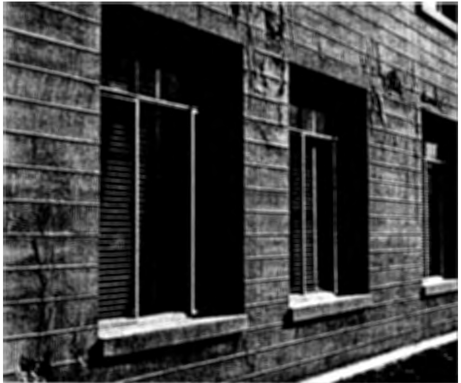
Much of the Pentagon's exterior concrete is in disrepair.
