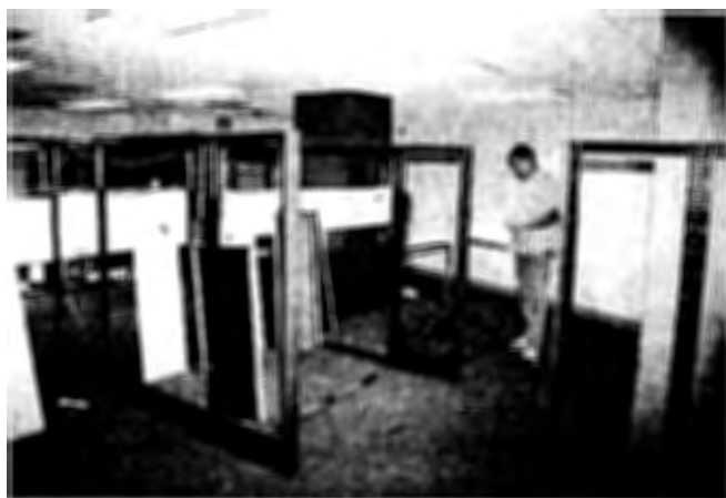
Assembling new partition walls in the basement
