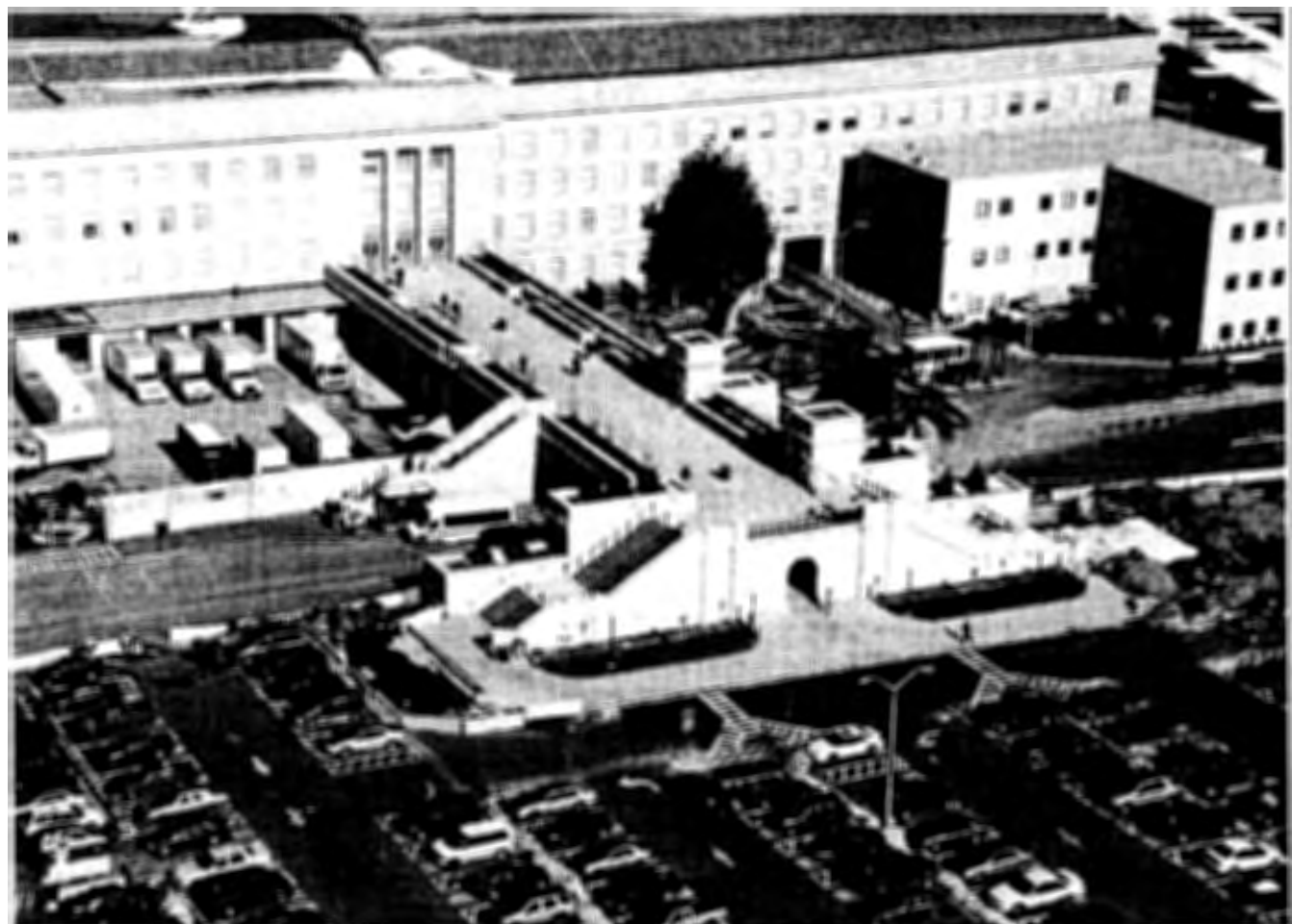
A close aerial view of the pedestrian bridge at Corridor 2. Two elevators in the bridge provide access for persons with disabilities.
