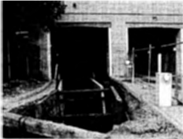
A trench was excavated for a new 36-inch chilled water line.
