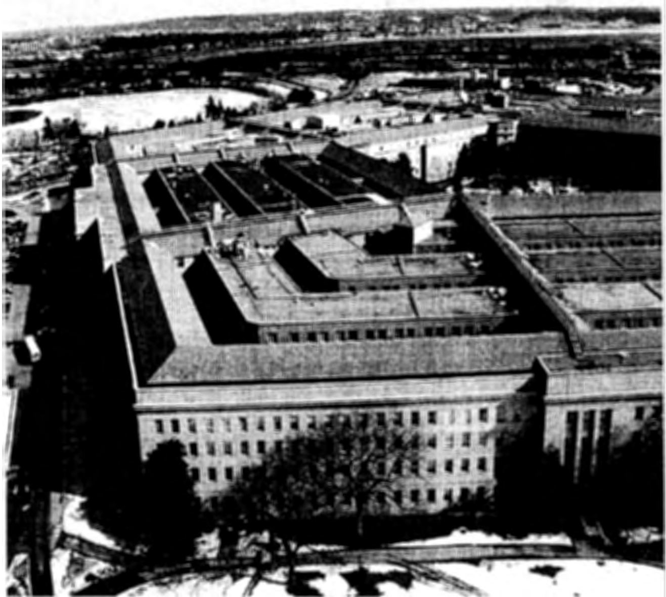
Aerial view of the Pentagon looking over Wedges 2 (foreground) 3, 4. Wedges 2 through 5 are currently being planned as a single acquisition, with phased construction. The objective is to realize cost savings with one prime contractor through the benefits of a true partnering environment.
