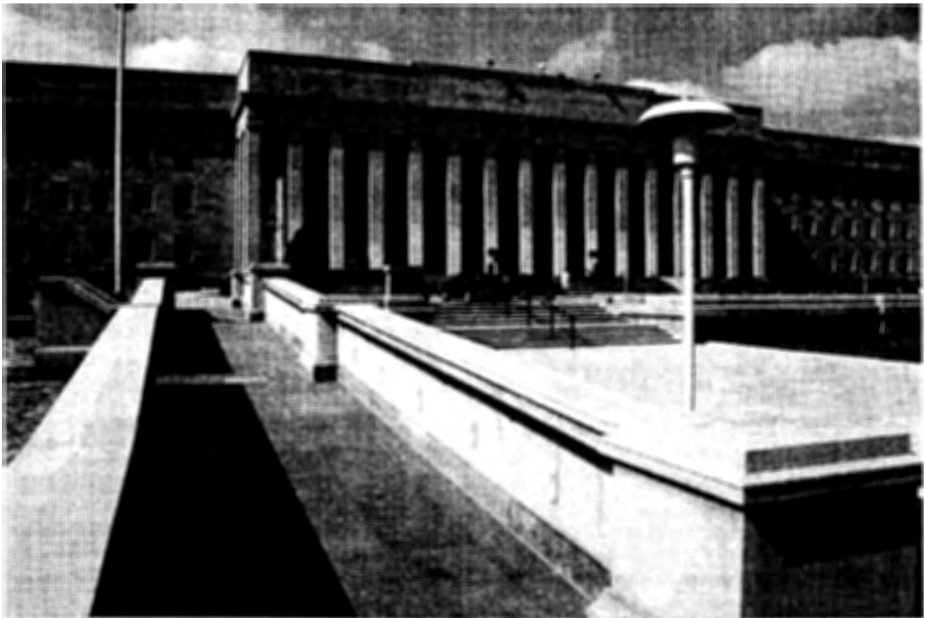
A new wheelchair ramp for persons with disabilities marked the first time in 55 years that limestone had been added to the Pentagon. The new stone was obtained from the Indiana quarry where the original limestone was cut for the Pentagon to match the color and texture of the River Terrace facade. Another ramp lies on the opposite side of the parade field.
