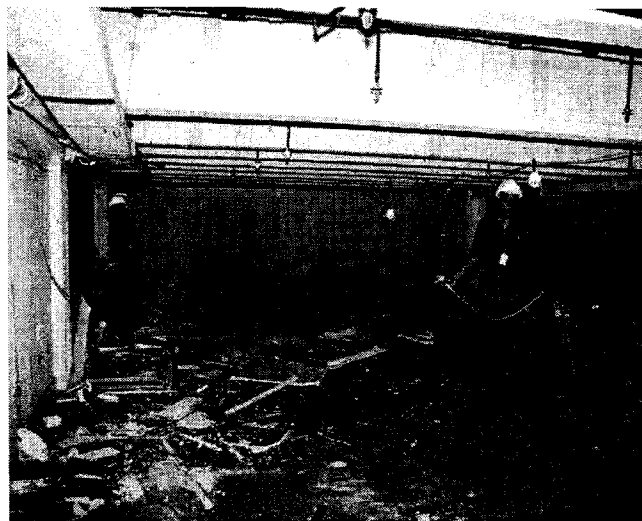
To minimize dust, a worker sprays water on debris as it falls during the demolition process.
