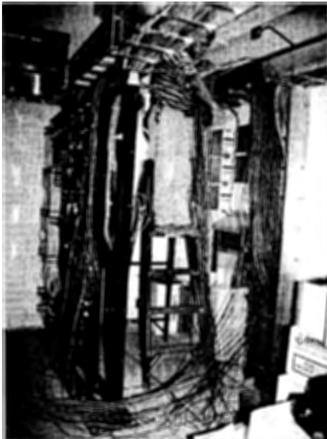
An IT specialist installs data wiring harnesses inside a new telecommunications closet in the Pentagon's basement.
