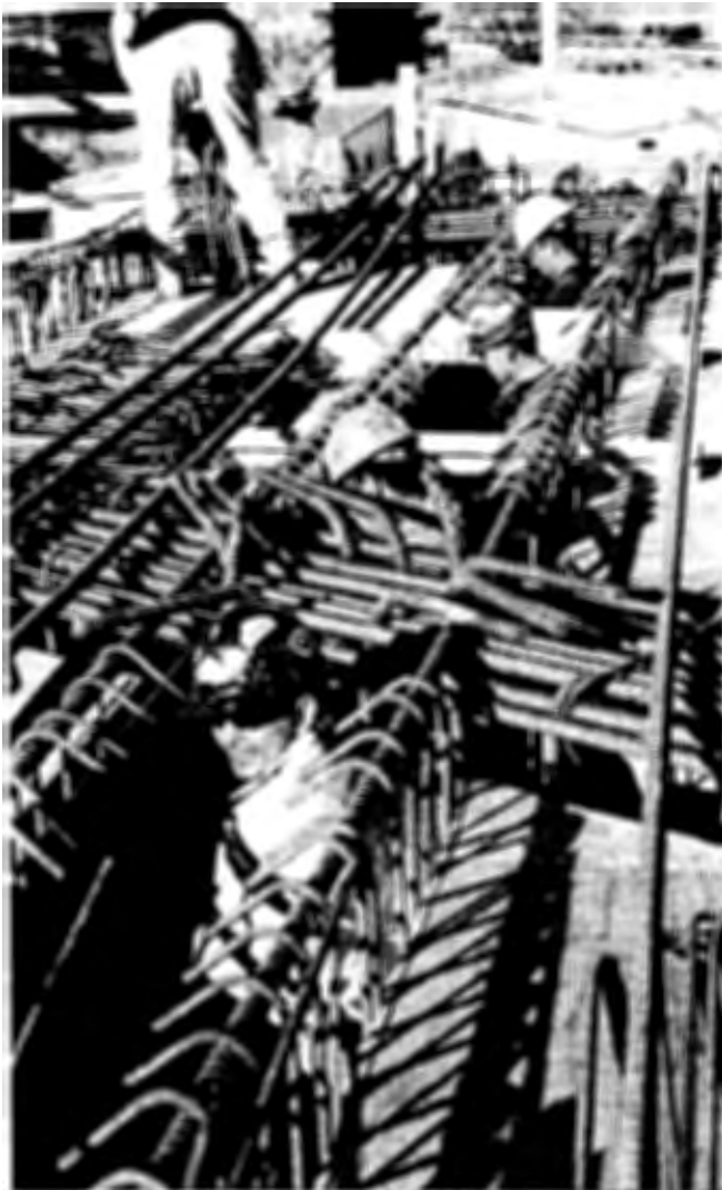
Workers install a complex system of roof beams and slabs for the Remote Delivery Facility.
