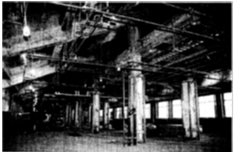
Steel beams now occupy an area where ramps once traversed all five floors in Wedge 1. The area will become office space.
