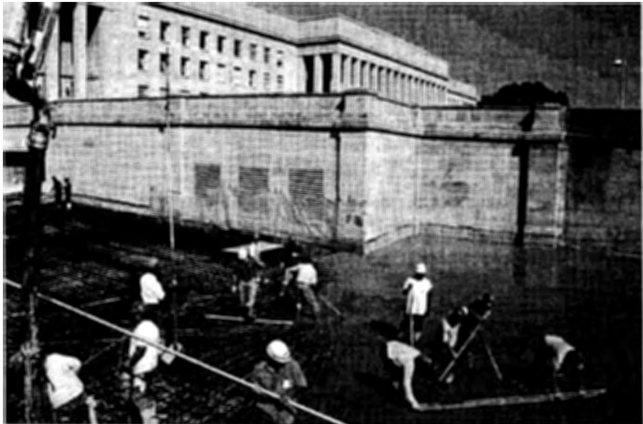
A crew readies concrete for the curing process. The site is directly above renovated space and will serve as a parking area adjacent to the new clinic entrance.
