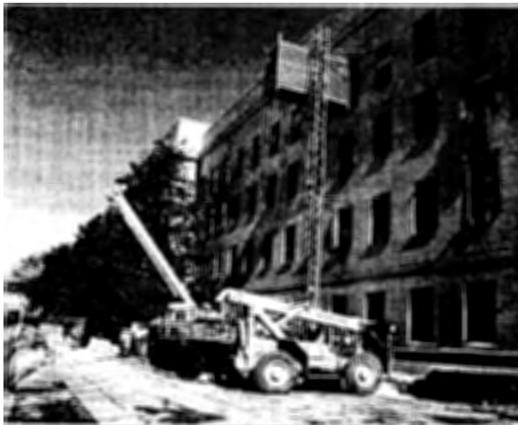
An external hoist facilitates the safe removal of hazardous materials from Wedge 1 by eliminating the need to transport it through the Pentagon.
