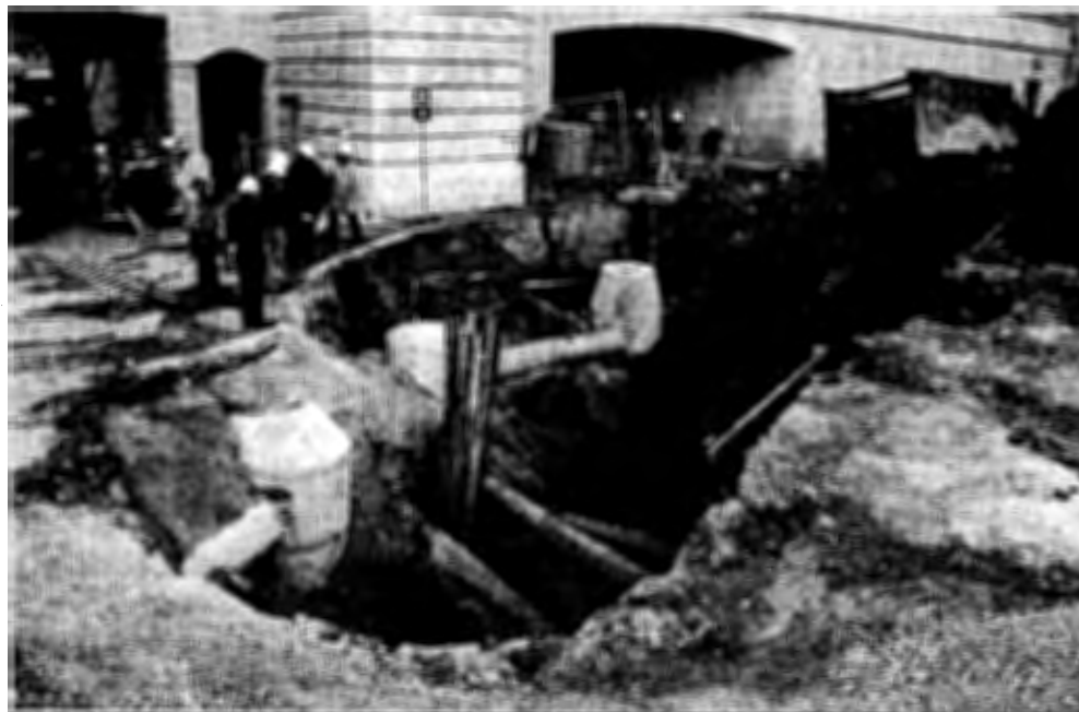
Installation of the new chilled water line.
