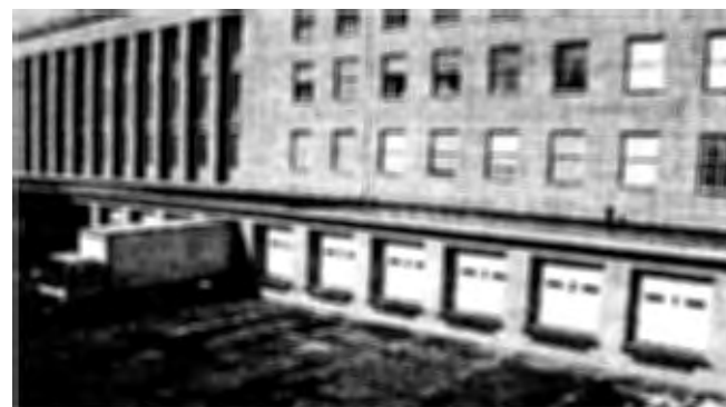
The South Terrace loading dock as it appeared in February 2000. Eventually, all trucks will be diverted to a new Remote Delivery Facility being constructed north of the Mall Terrace.
