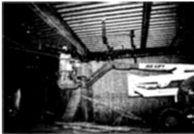
Under a new cafeteria floor between rings in Wedge 1
