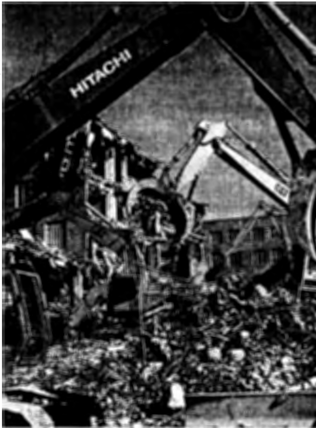
November 5, 2001 - Demolition work progresses 24 hours a day, 6 days a week. Demolition was completed four weeks ahead of an aggressive eight week schedule.
