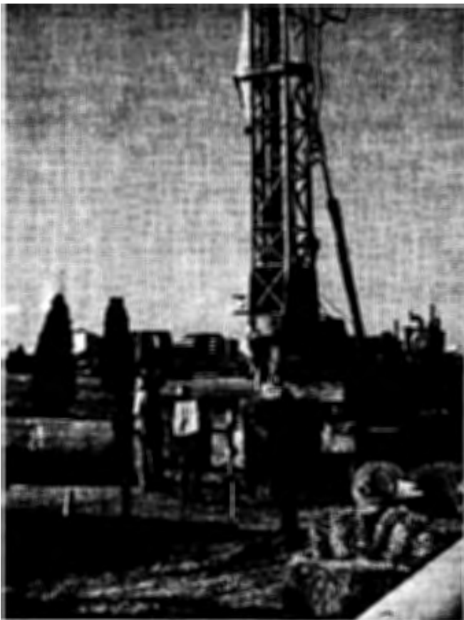
Preliminary drilling for the water intake line along the banks of Boundary Channel Lagoon. Workers will drill about 70' into the earth, where the intake lines will be placed and tunneled to the H&RP.
