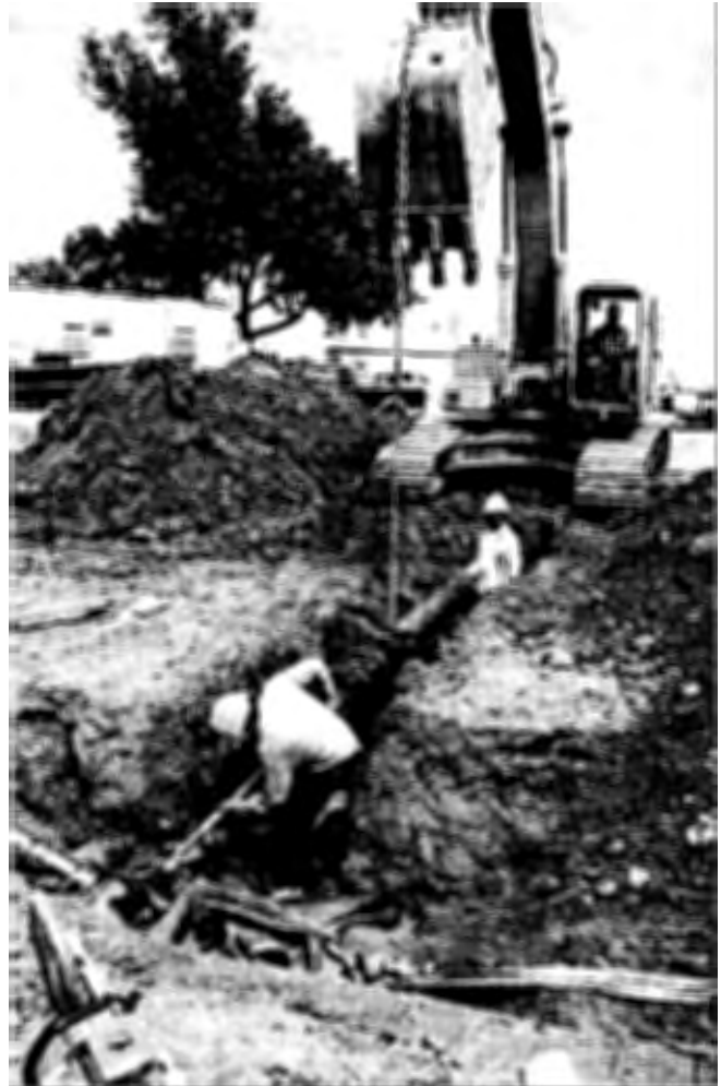
Workers preparing for the installation of new Chilled Water Line Feeders.
