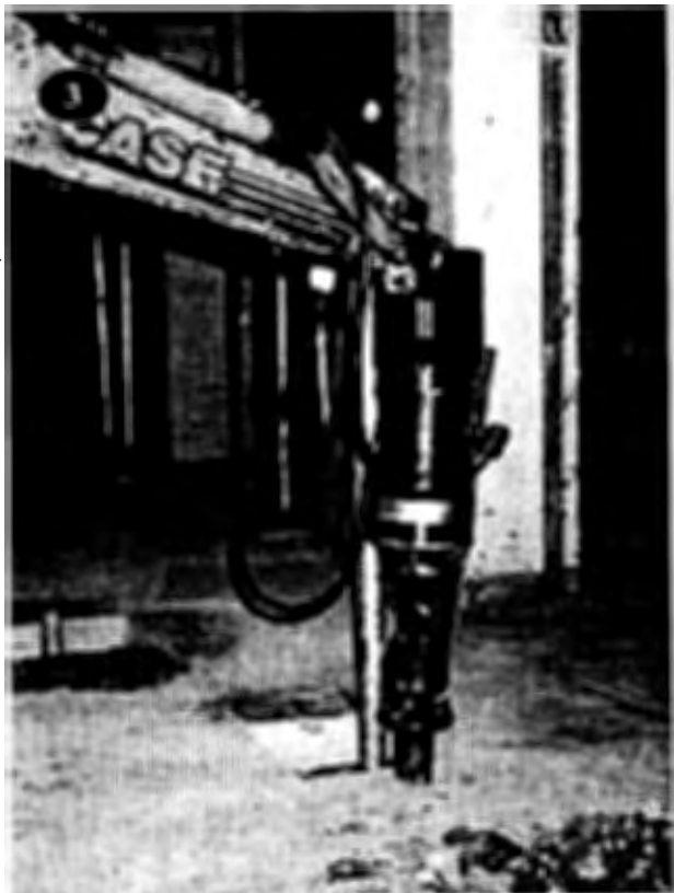
Preparing the helical screwed piles. A worker first cuts out a rectangular area in the floor (1), to mark the area where the screws (2) are to be machine driven (3). The slabs are placed on top of the helical screws.
