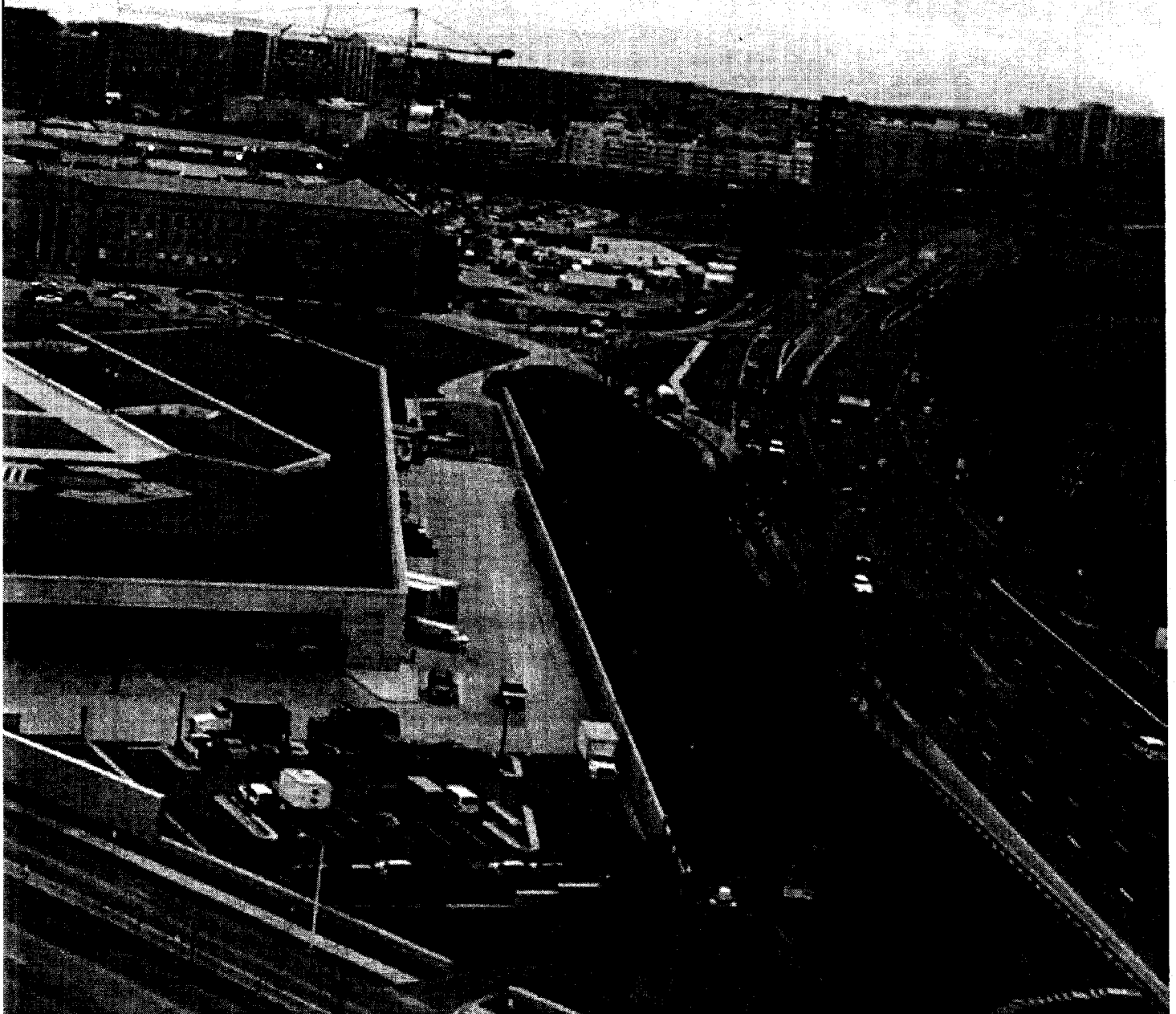
The location of the Remote Delivery Facility enhances Pentagon security by diverting all delivery vehicles from the surrounding highways away from the building.
