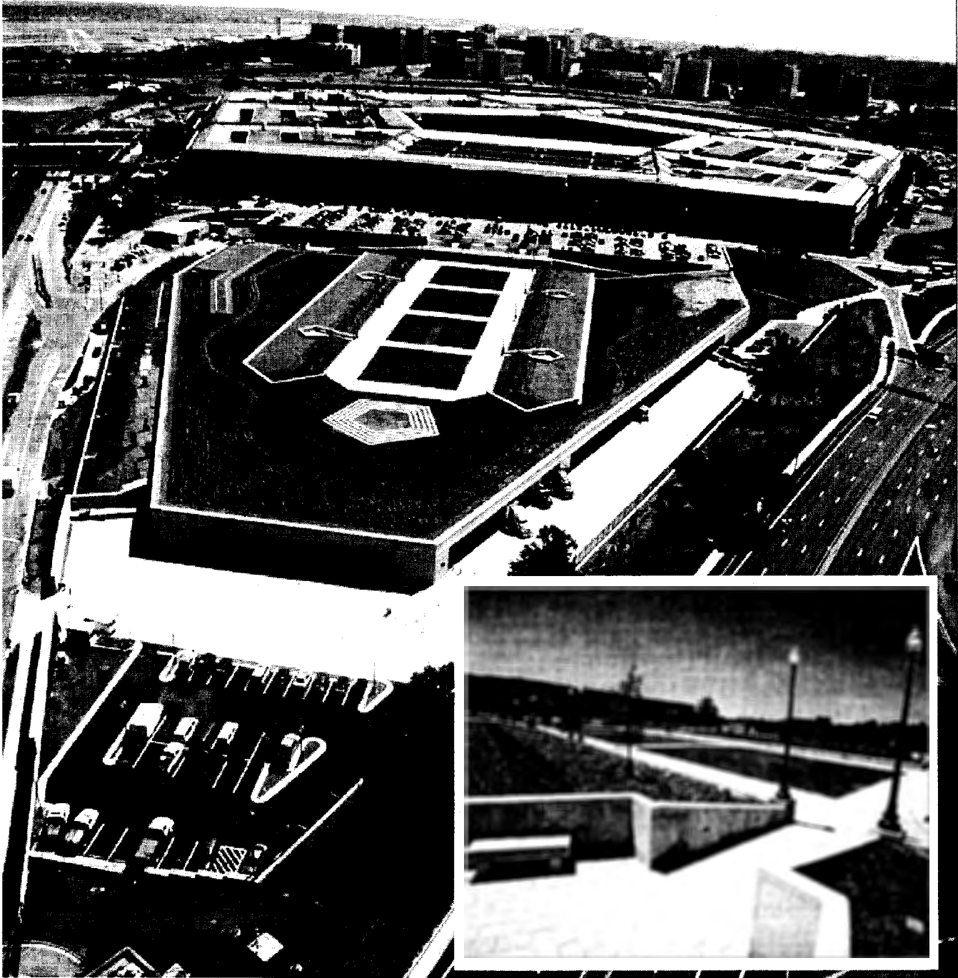
The Remote Delivery Facility is located adjacent to the Pentagon's Mall Terrace between Rt. 110 (left) and Rt. 27 (right).
