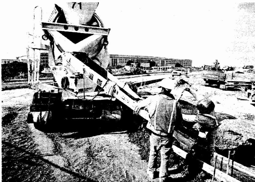
The September 11 attack placed a new emphasis on the need for security. Work on the Metro Entrance Facility Project, a security-driven initiative, was already well underway. The Pentagon Transit Center opened for business on December 16, 2001.
