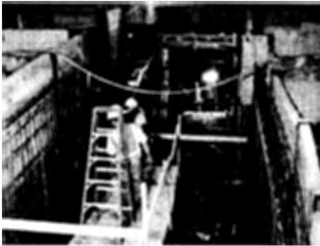
Above, excavation work progresses on the General Purpose Switch Room Tunnel, a project essential to the modernization of information and telecommunications in the Pentagon. Below, the existing A-ring steam tunnel has been cleared of all old utilities. The metal racks will be used to shelve conduits for data cable and wiring.
