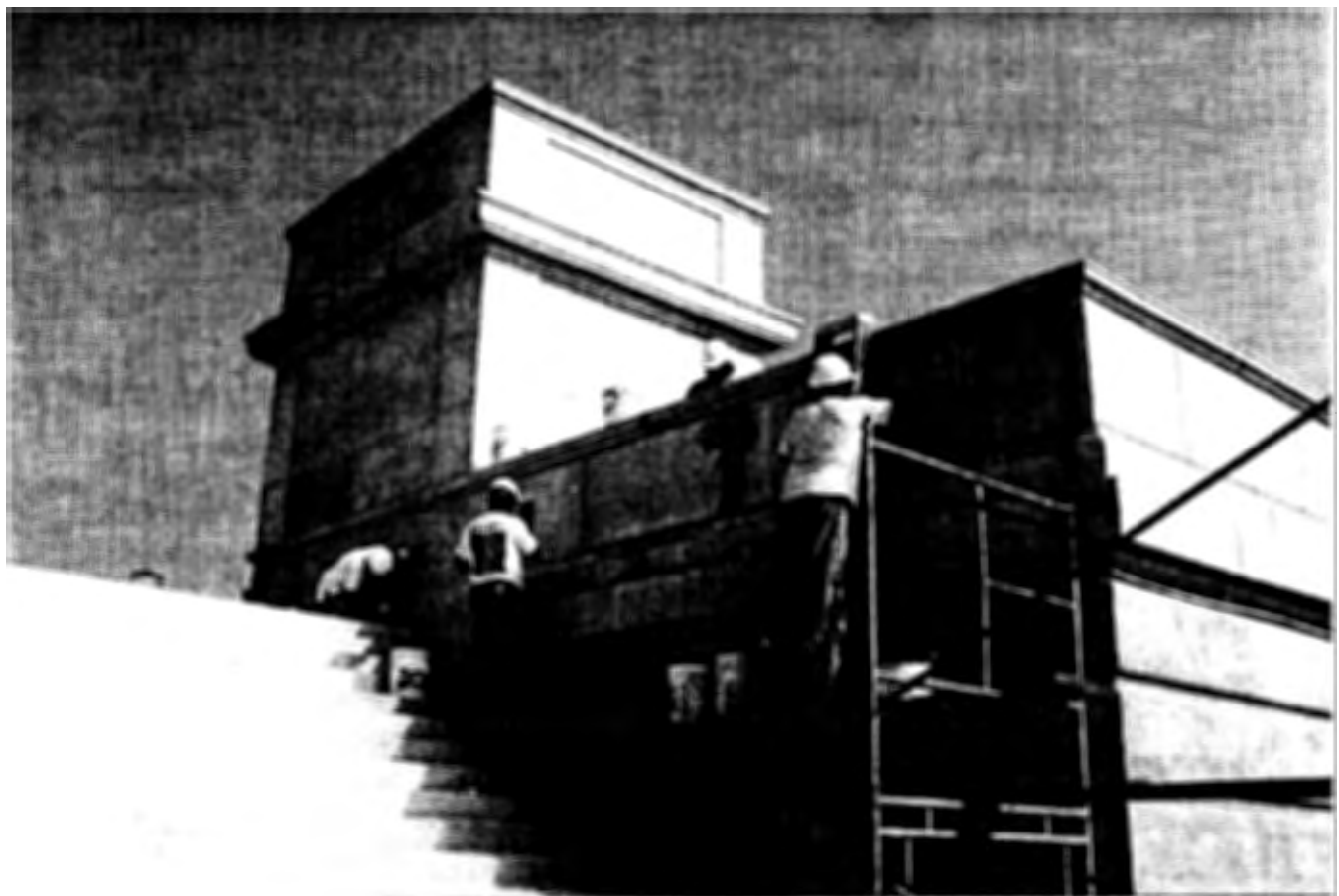
The new limestone cladding used on the South Terrace Pedestrian Bridges was mined from the same vein of stone in Indiana used during the Pentagon's original construction in 1941.
