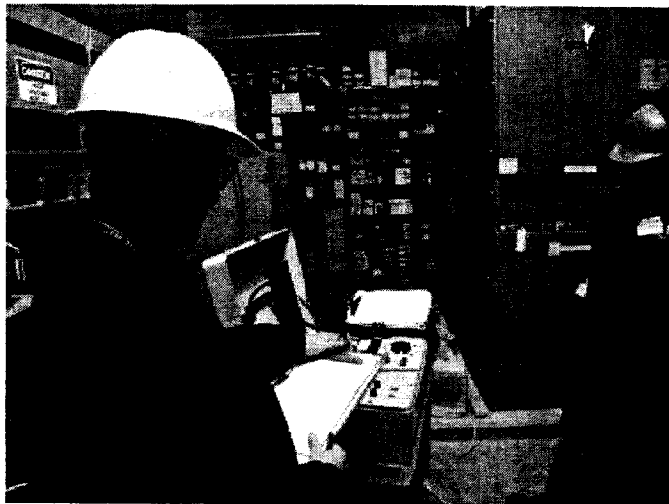
Testing begins on a Wedge 1 electrical vault. The original vault was destroyed in the September 11 attack. This particular test measures the integrity of the wiring that feeds the vault.
