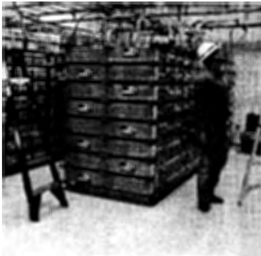
Back up battery installation in Wedge 1
