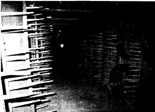
Above, excavation work progresses on the General Purpose Switch Room Tunnel, a project essential to the modernization of information and telecommunications in the Pentagon. Below, the existing A-ring steam tunnel has been cleared of all old utilities. The metal racks will be used to shelve conduits for data cable and wiring.
