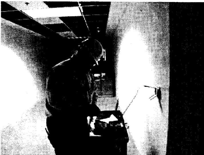
A contractor testing and calibrating the air flow in the Wedge 1 HVAC ducts.
