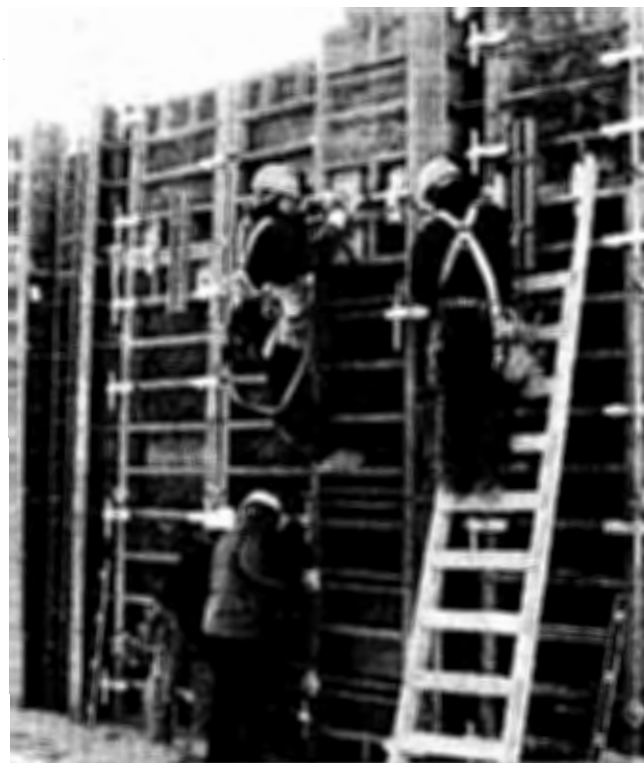
The E-ring wall begins to rise on the exterior of the Phoenix Project.
