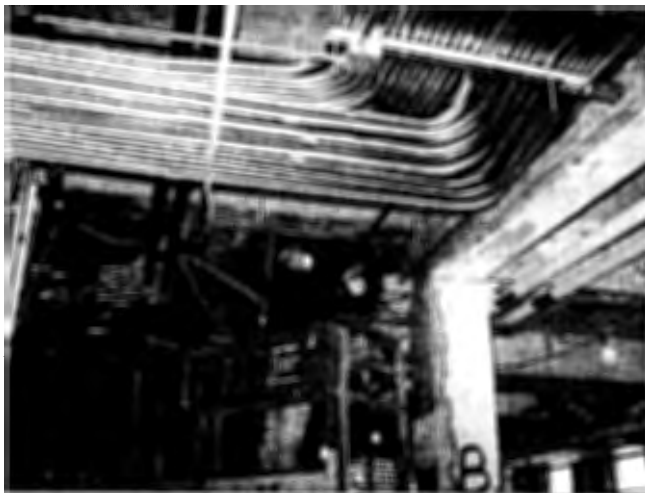
Before demolition in Wedge 1 could begin, temporary utilities and communication lines had to be installed.
