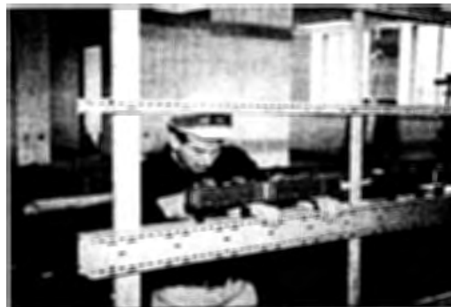
A worker installs the spine-wall for office systems furniture in Wedge 1. The IM&T lines run through the spine-wall to connect up to four separate workstations.
