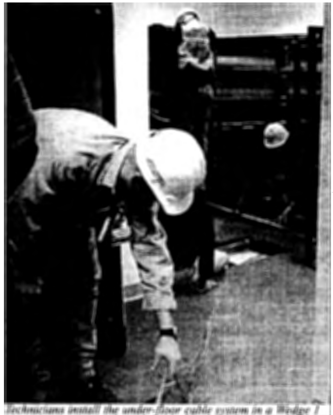
Technicians install the under-floor cubic system in a Wedge 1 tech facility.
