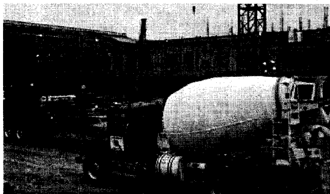
January 15, 2002 - A concrete truck arrives on-site to continue the pouring of the E-ring wall.
