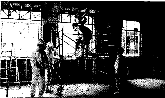
Abatement of windows in Wedge 1.
