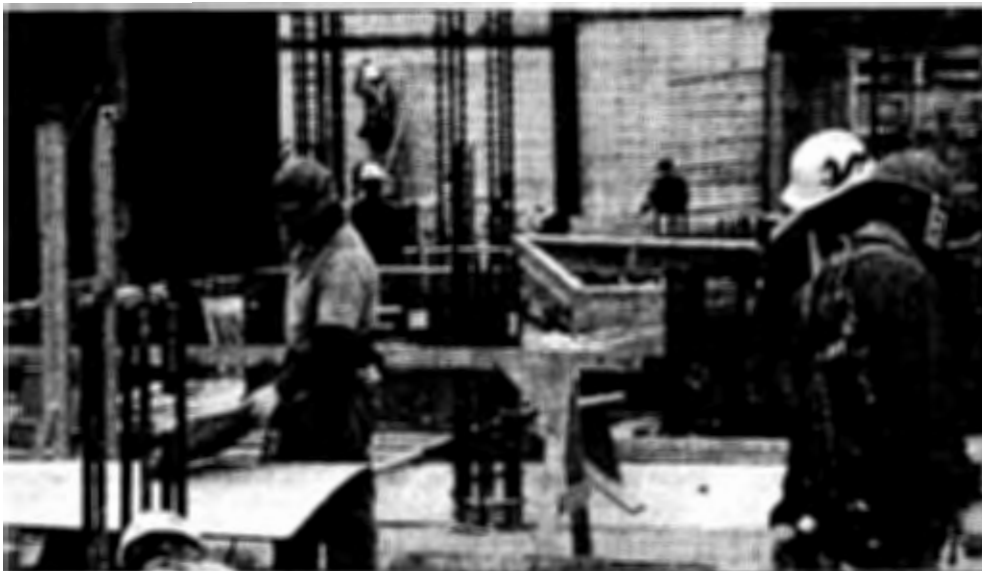
Workers place formwork on the third floor of the Phoenix Project. The necessity to construct a safer, stronger Pentagon is the driving factor behind the advanced schedule.
