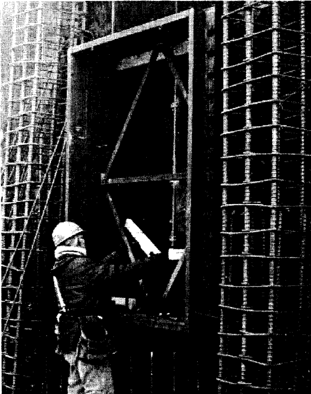
December 28, 2001 - Installation of the first E-ring window frame.
