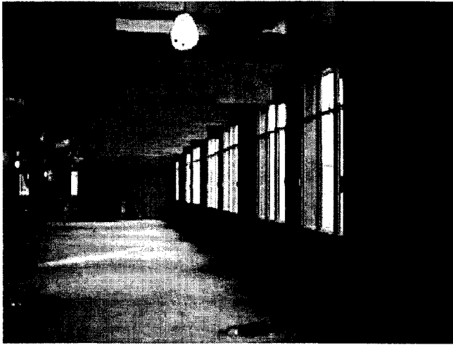
These photos show Wedge 2 areas on the fourth floor, where demolition has been completed and core and shell work has begun. In the top photo, new windows have been installed. Below, a view of some initial ductwork.
