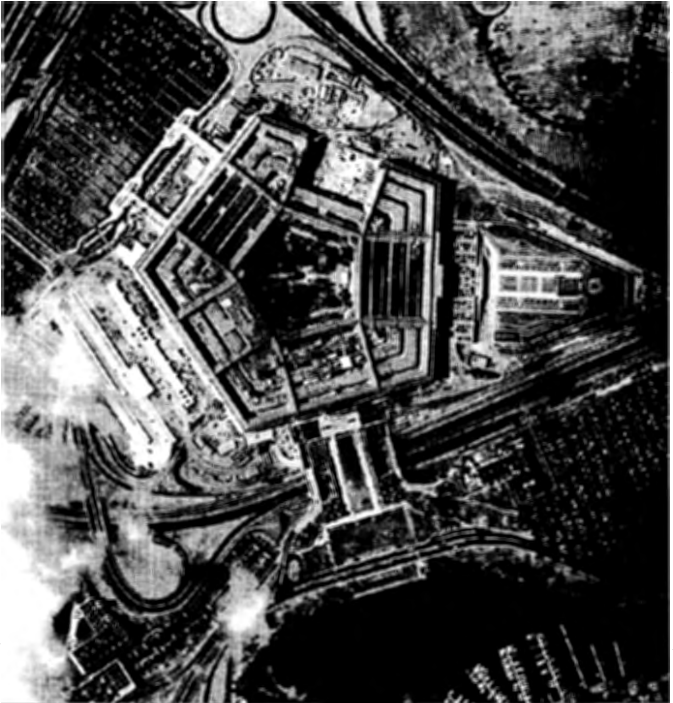
An aerial view of the Pentagon, November 20, 2001, one day after demolition was completed on the Phoenix Project.
