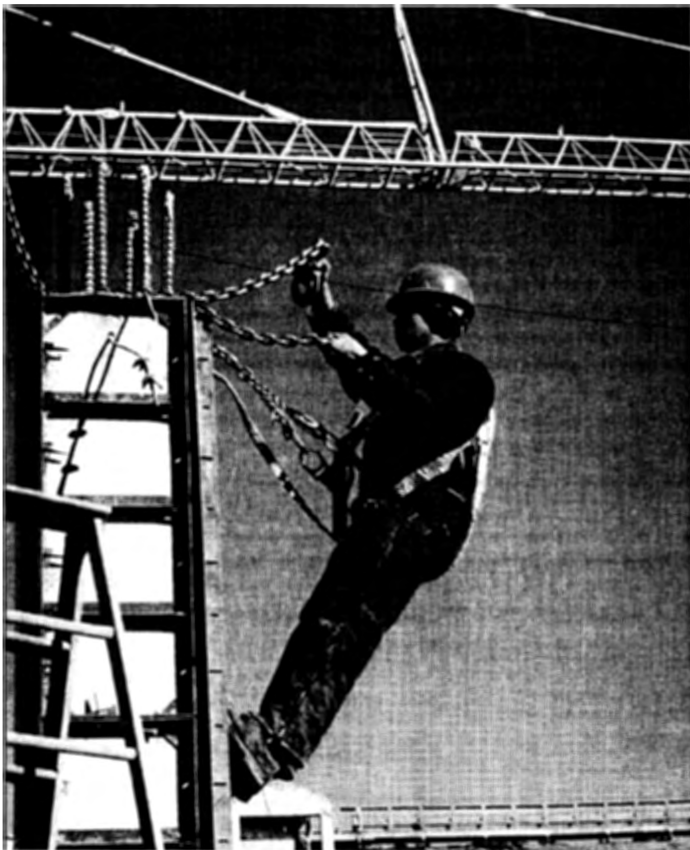
A worker on the Phoenix Project erects formwork before placing the concrete for a structural support column.
