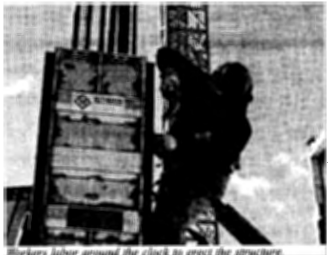
Formwork for a structural column is secured in place.
