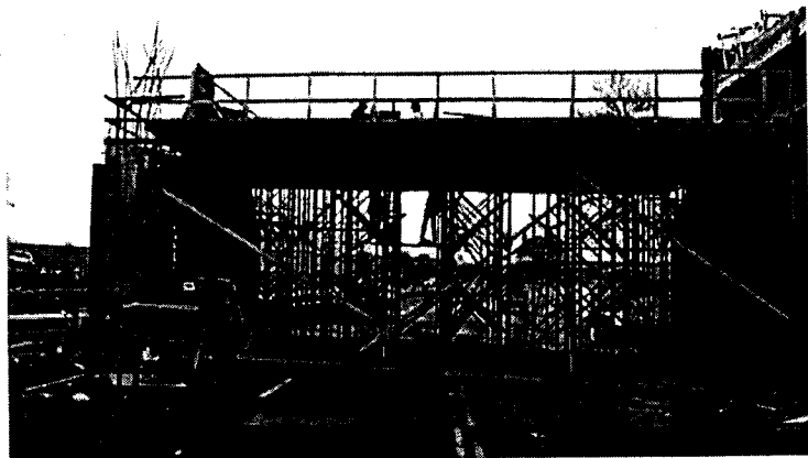
River Terrace Vehicle Bridge Under Construction
