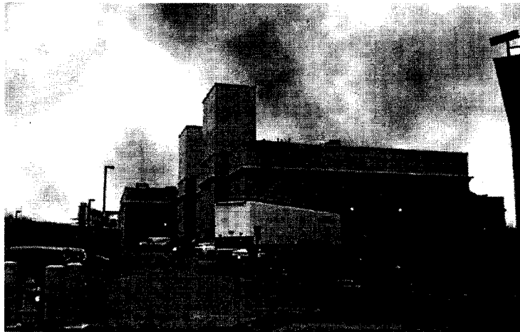
New Heating & Refrigeration Plant
