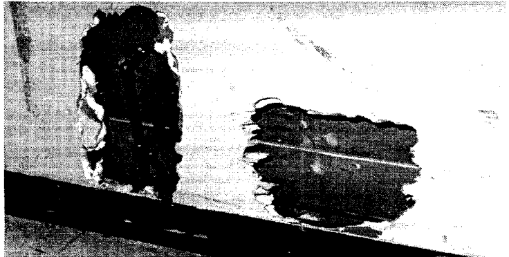
Typical Plumbing Problems
