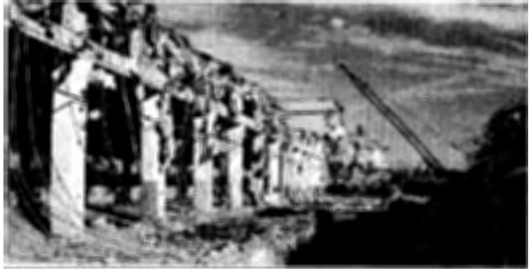
Old Heating & Refrigeration Plant Being Demolished
