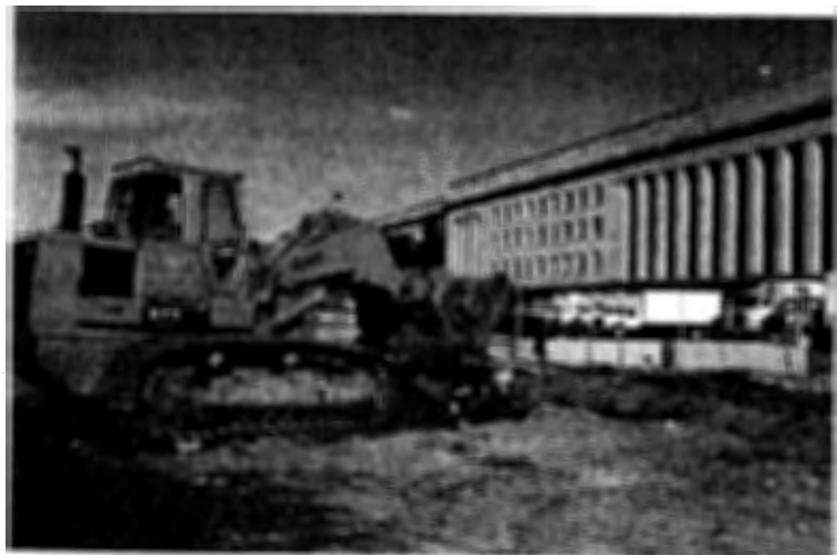
Beginning of Roadway Preparation
