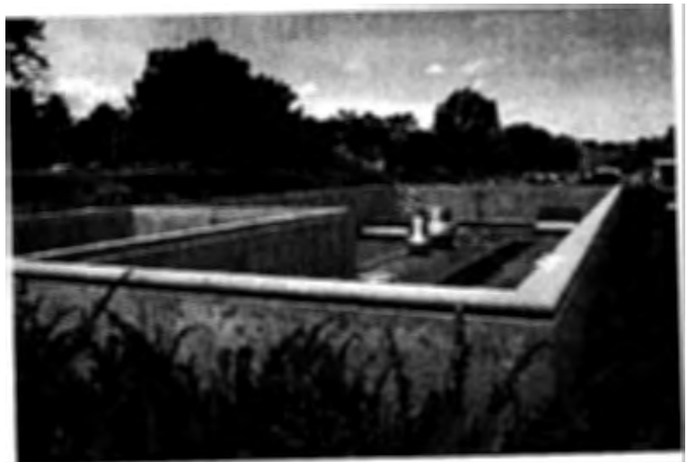
Completed Sewage Lift Station with Landscaping
