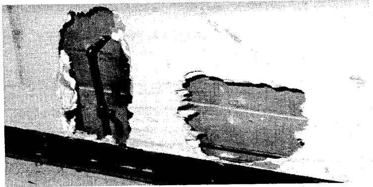
Typical Plumbing Problems in Walls
