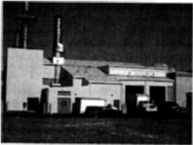
Completed Classified Waste Incinerator Plant
