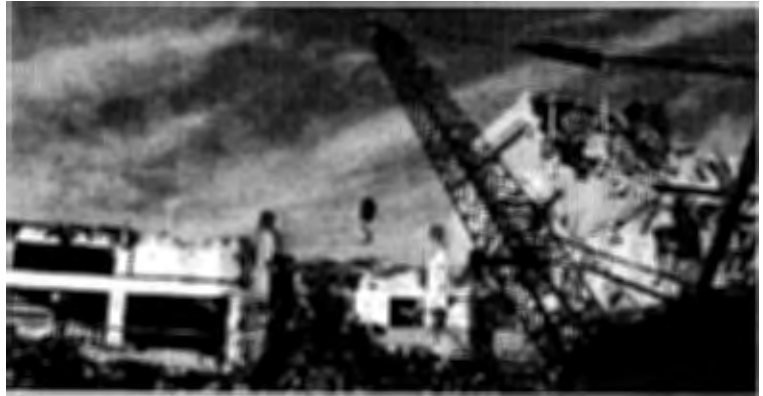
Old Heating & Refrigeration Plant Being Demolished
