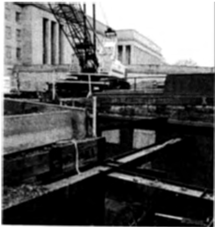
Foundations - Under Construction
