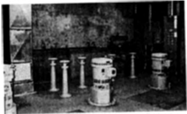
Completed Sewage Lift Station Interior
