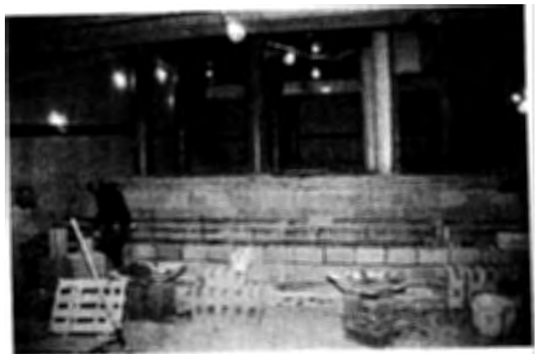
Construction of Ramp
