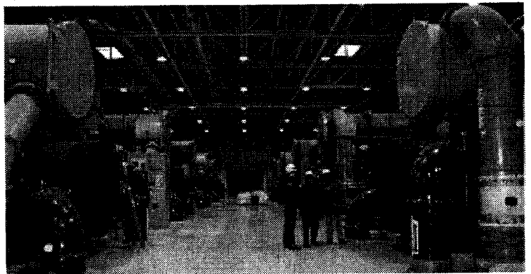
Completed New Heating & Refrigeration Plant (Chillers)
