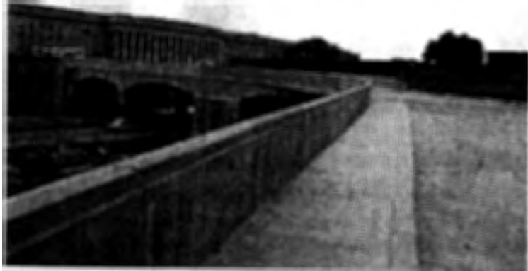
Completed Sidewalk and Wall
