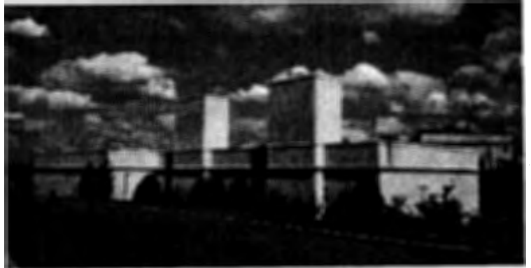
Completed New Heating & Refrigeration Plant
