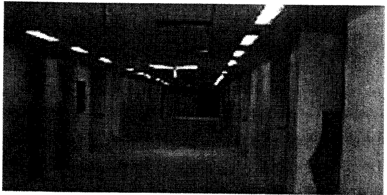
Corridor #8 - Under Construction
