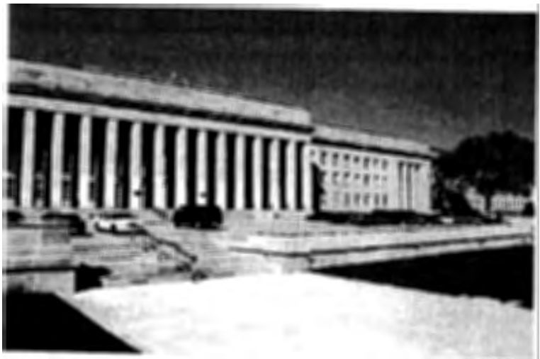
Completed Steps, Walk, and Planters
