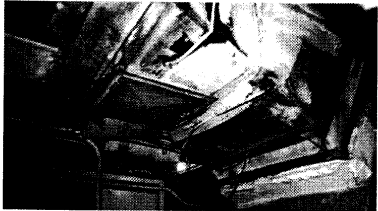
Deteriorating Heating, Ventilation, and Air Conditioning (HVAC) Ductwork.
