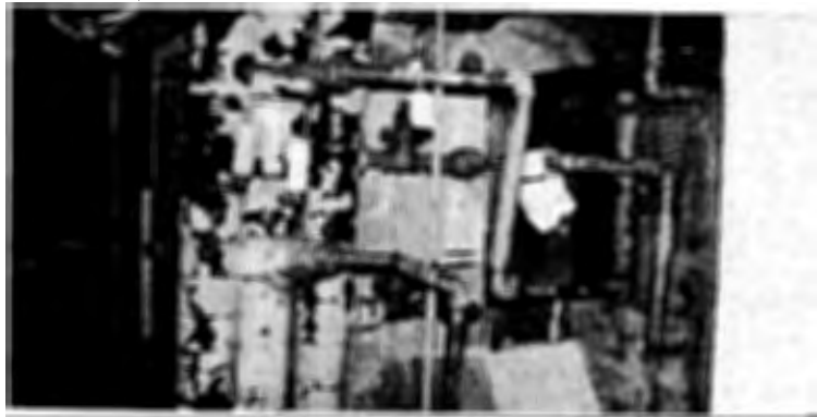
Typical Existing Asbestos Piping Insulation
