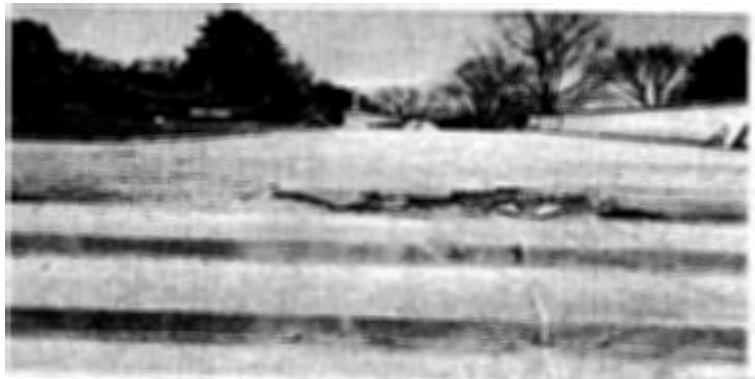
Typical Deterioration of River Terrace Stairs
