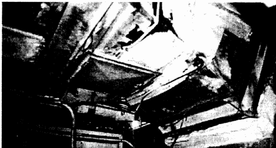
Figure 3 Deteriorating Heating, Ventilation, and Air Conditioning (HVAC) Ductwork
