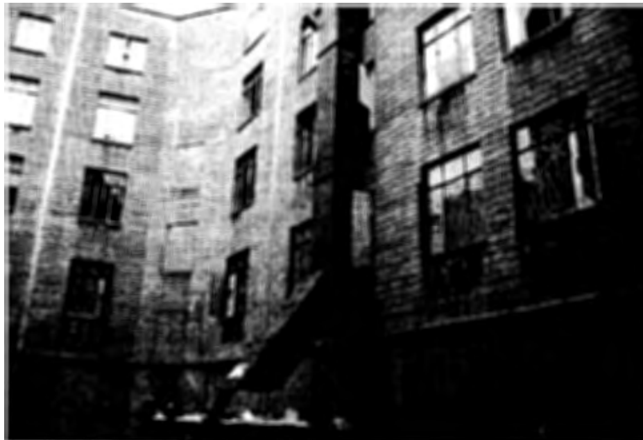
Figure 55 Trash Chutes Installed on A/E Drive for Top Four Floors
