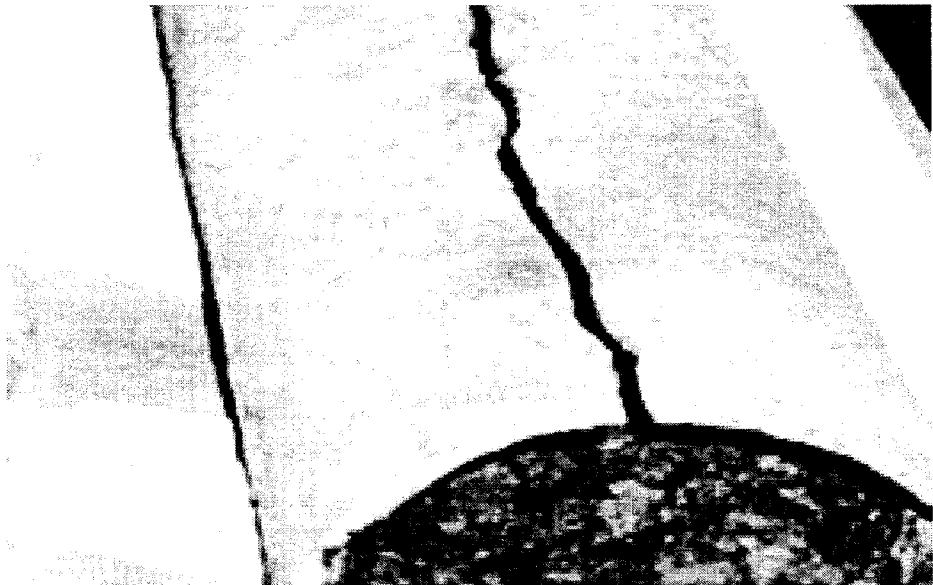
Figure 68 Vertical Sanitary Pipe Split from First to Fourth Floor
