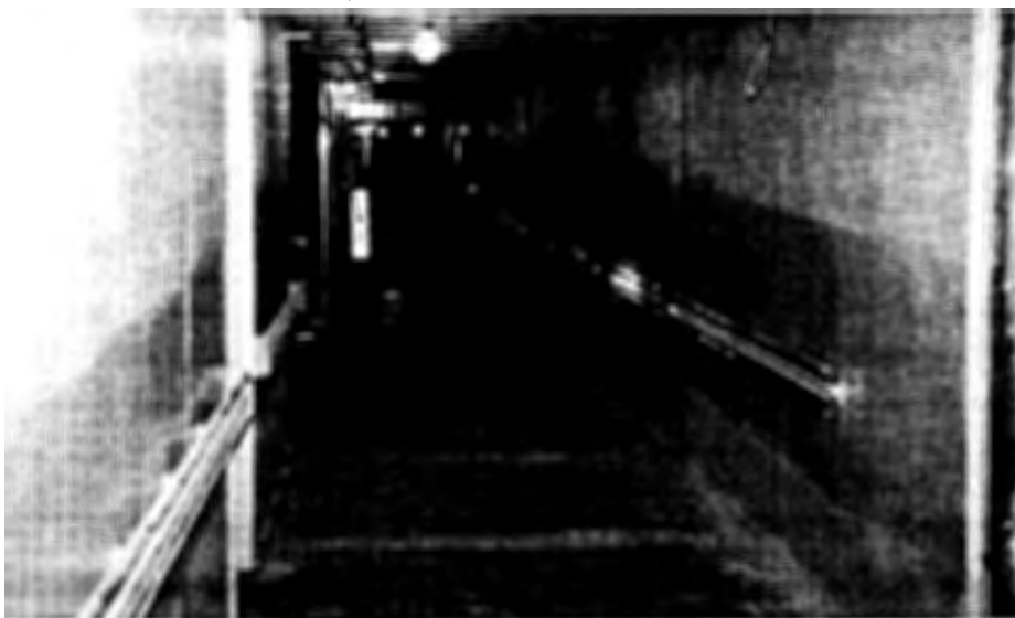
Figure 52 Completed Guardrails Will Protect Walls from Gurneys
