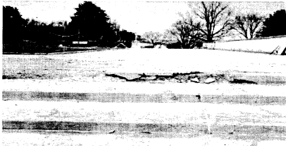
Figure 75 Typical Deterioration of River Terrace Stairs
