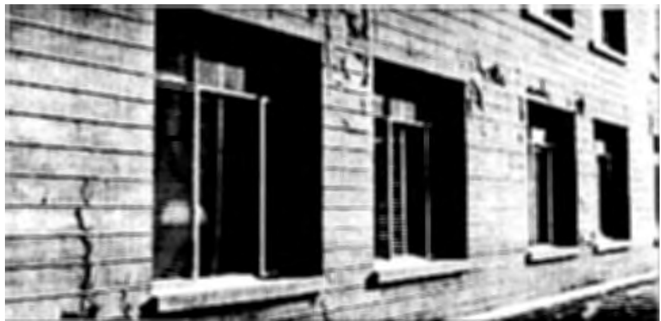
Figure 73 Typical Exterior Walls in Light Wells Needing Repair
