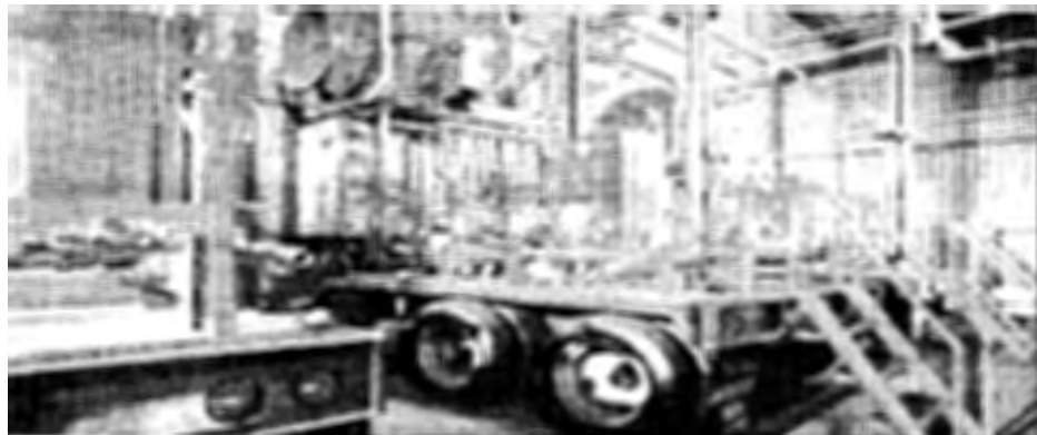
Figure 80 Portable Rental Boilers Used in Old HR&P
