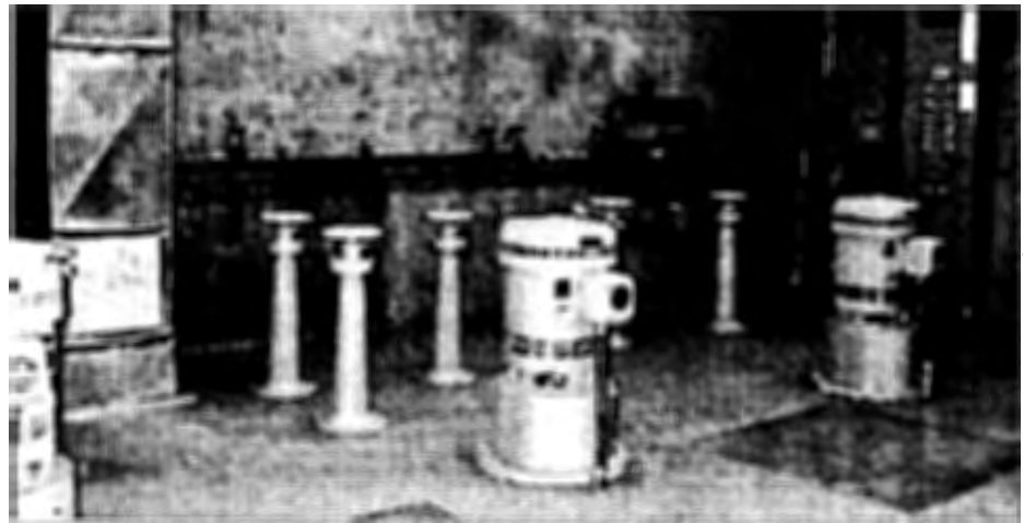
Figure 31 Interior View of Sewage Lift Station
