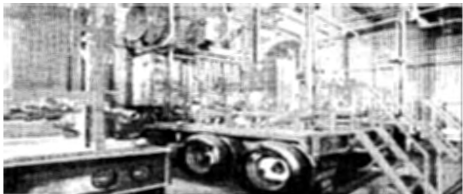
Figure 80 Portable Rental Boilers Used in Old HR&P
