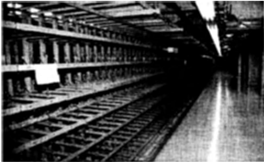
Figure 21 The Main Distribution Frame in the General Purpose Switch Room (Construction Complete, IM&T Installation Underway)
