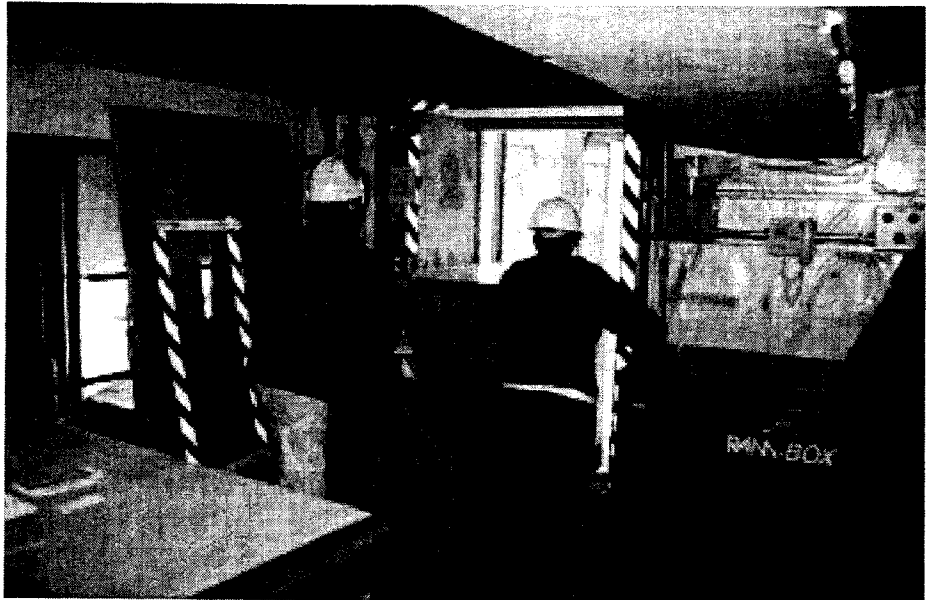
Figure 57 Wedge 1—Employees Push Hazardous Materials Onto An External Hoist
