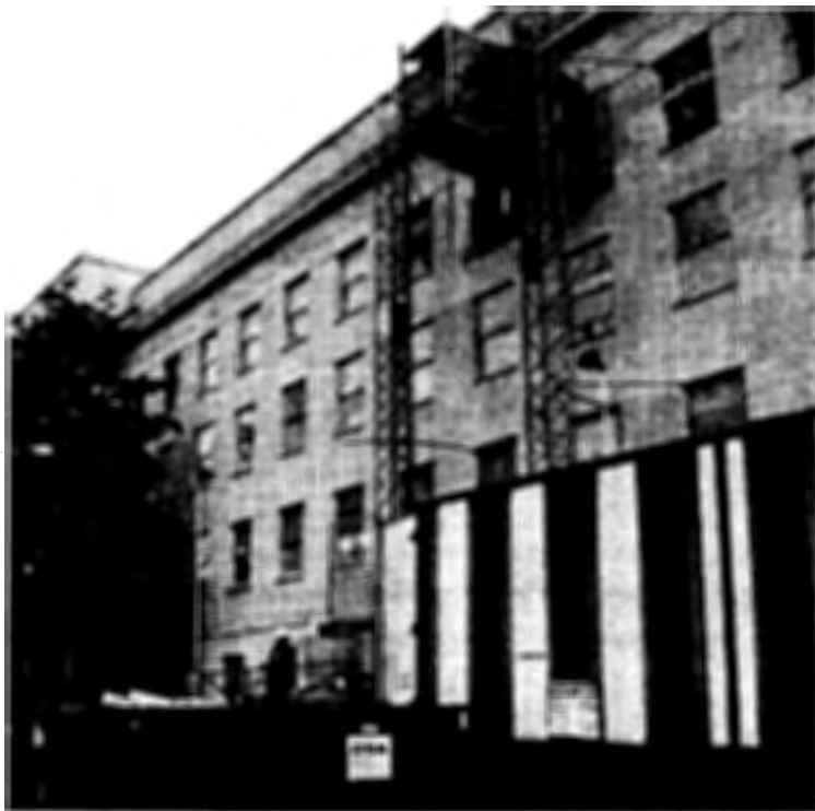
Figure 56 Wedge 1—An External Hoist Allows for the Safe Removal of Hazardous Materials
