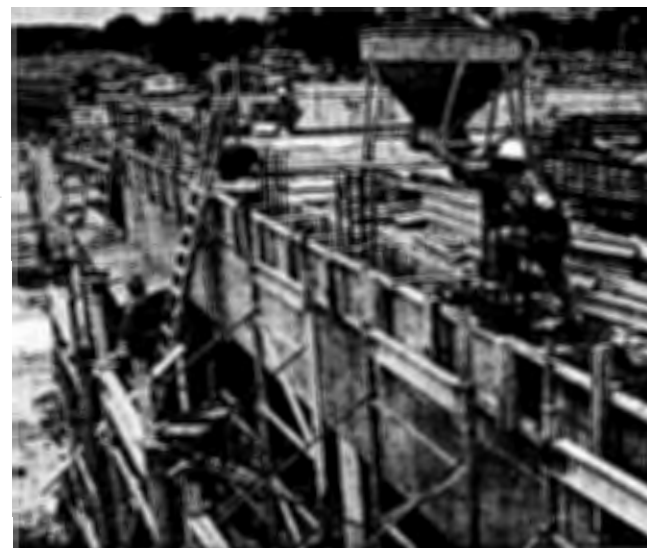
Workers place concrete on the roof of the Remote Delivery Facility.
