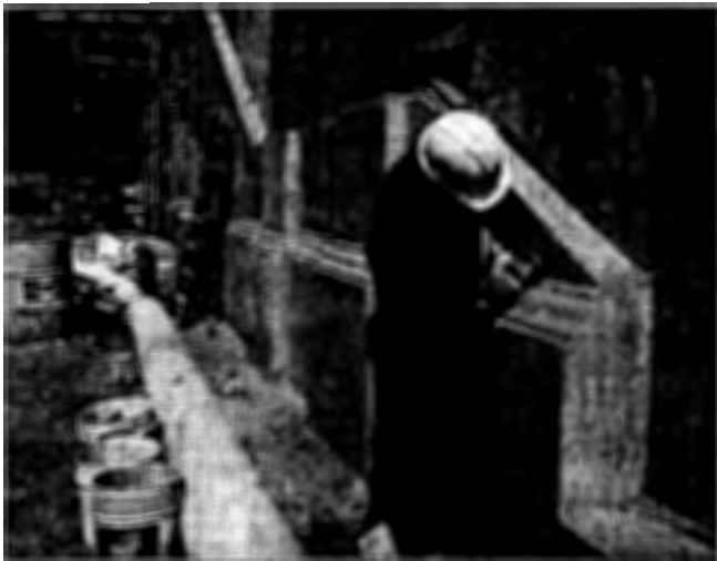
Concrete is "sculpted" on the outer face of the South Terrace Pedestrian Bridge at Corridor 3 to match the architectural molding of the Pentagon.
