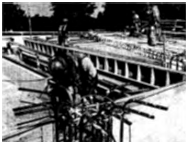
Worker ties rebar for a structural column of the Remote Delivery Facility.
