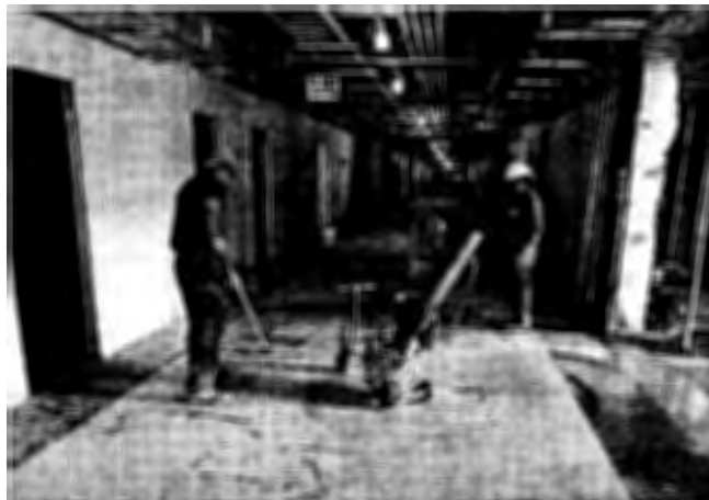
The terrazzo floor installation in Wedge 1 is part of core and shell construction. Terrazzo was selected as a floor covering in high traffic areas because of its superior life-cycle cost.
