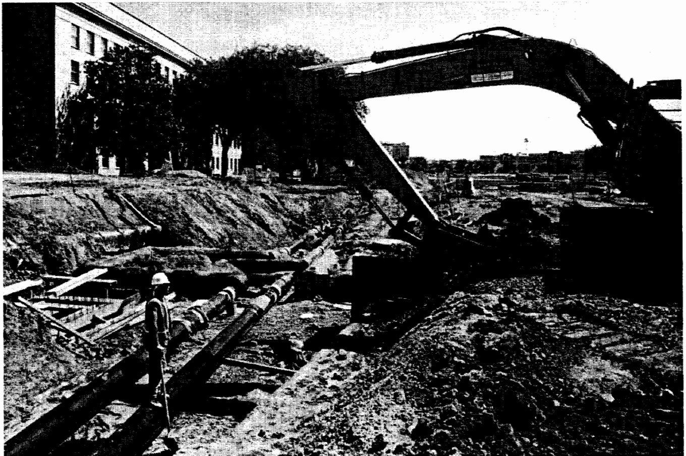
New chilled water lines will improve the reliability of the Pentagon's cooling systems.
