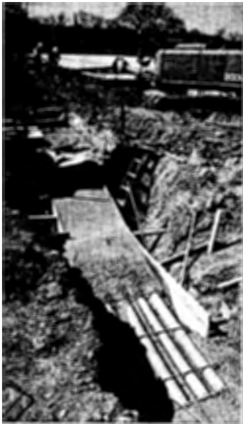
New information and telecommunications trench being completed on the Heliport side of the Pentagon.
