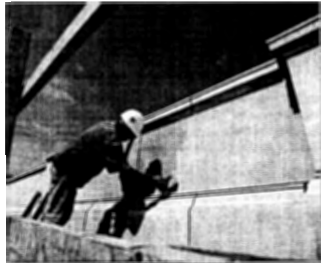
A worker washes new limestone on the South Terrace Pedestrian Bridge at Corridor 3. Limestone for the bridge project was obtained from the same Indiana quarry that provided the Pentagon its limestone in 1942 to ensure a close match of texture and color with the existing facade.
