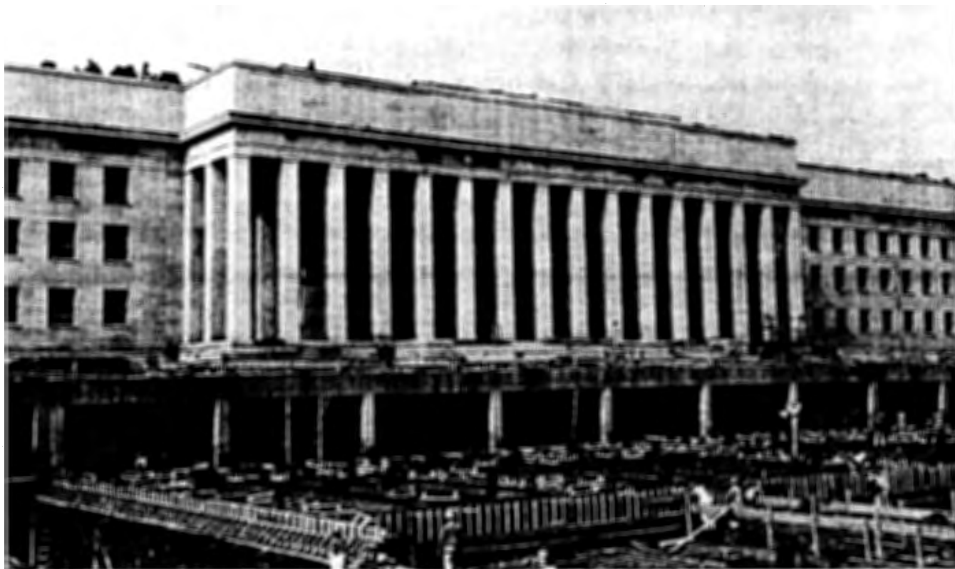
Work on the Pentagon's River Terrace progresses in 1942. Rather than backfill the entire site, engineers extended columns down to the existing grade. This resulted in a basement area below two fifths of the Pentagon.
