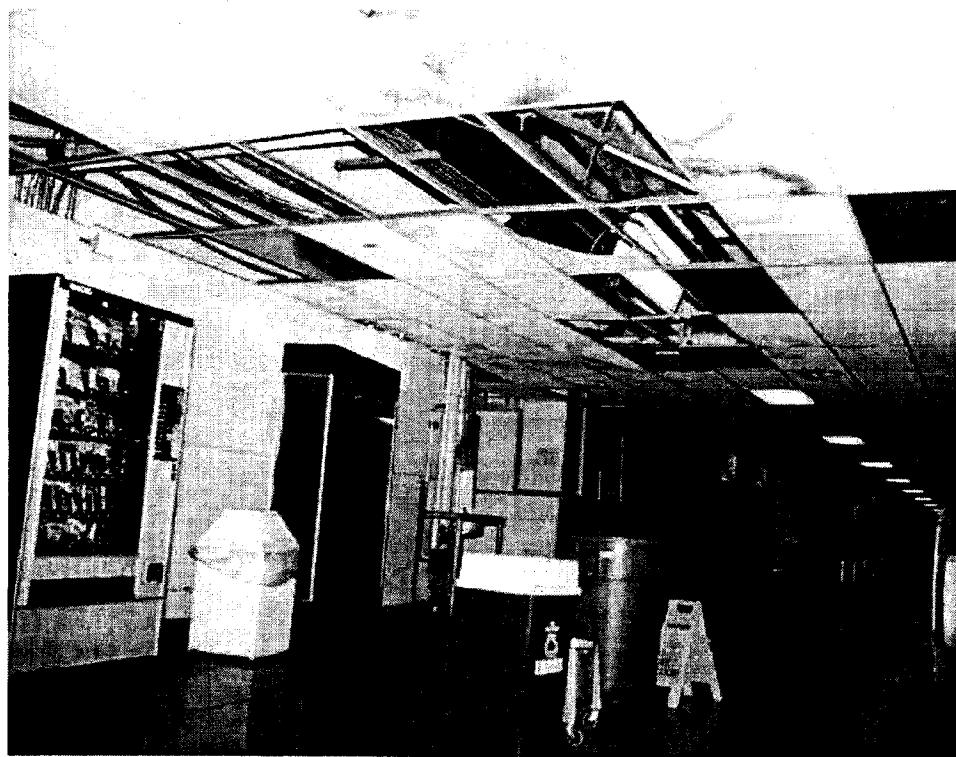
Garbage containers and buckets catch water leaking from pipes overhead in the Pentagon's basement. In addition to a sinking floor slab, water-stained ceiling tiles and dark corridors are commonplace in the lower levels of the building.
