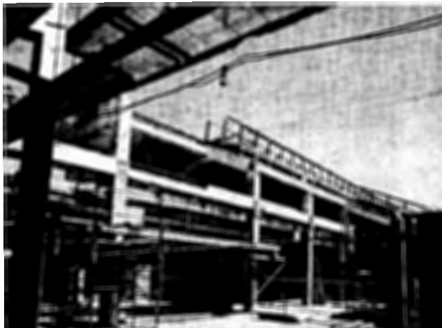
Some areas of the roof above Wedge 1 were exposed to clear the way for new elevator shafts.
