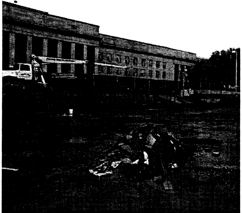
The entire River Terrace parking lot and a portion of the parade field were excavated to clear the way for waterproofing and repair to the area.
