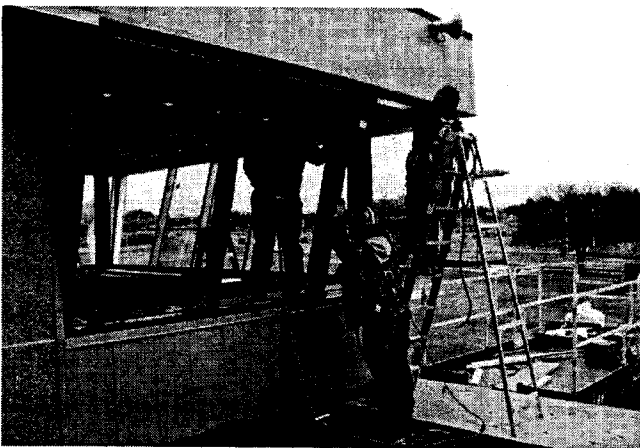
Window installation at the Heliport Traffic Control Tower.
