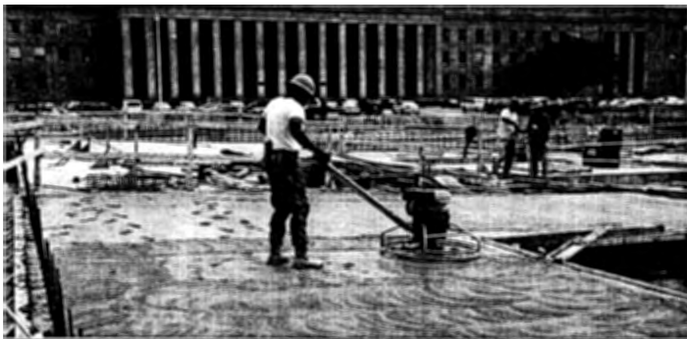
Worker finishes concrete slab on the roof of the Remote Delivery Facility.
