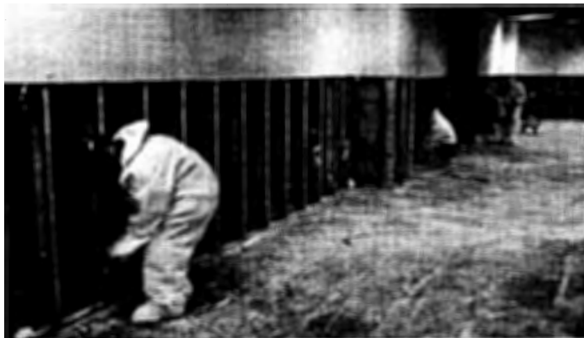
Dressed in Tyvek suits and wearing respirators, workers remove drywall that had been damaged when millions of gallons of water, from sprinkler heads and fire hoses, pooled in offices and corridors throughout Wedge 1 prompting the widespread growth of mold on walls and carpeting.
