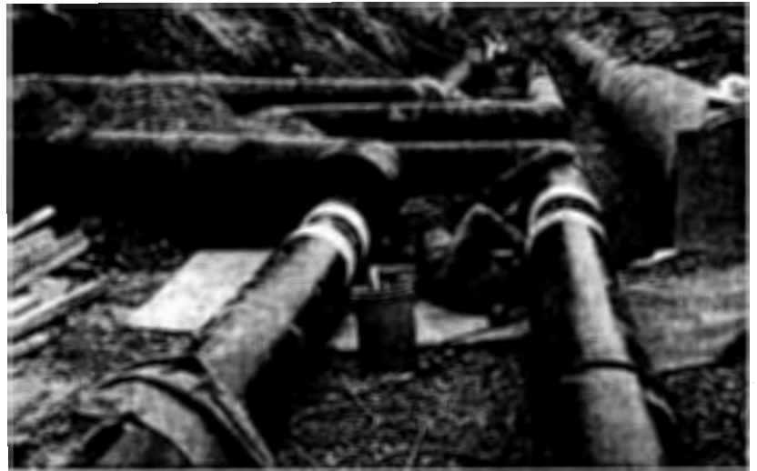
Worker welds joint of a new utility line.
