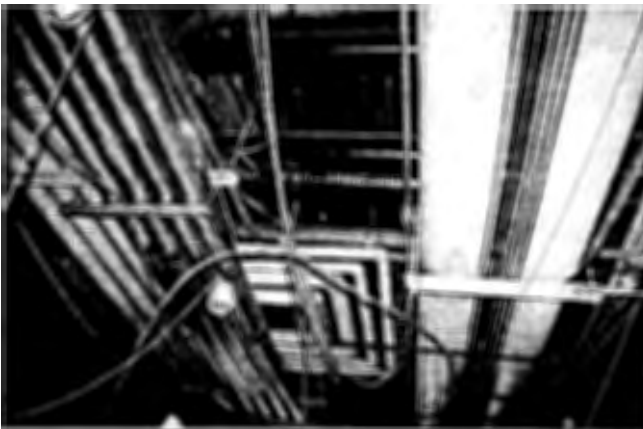
Undocumented pipes and conduits lined the ceilings in the Pentagon's basement and mezzanine.
