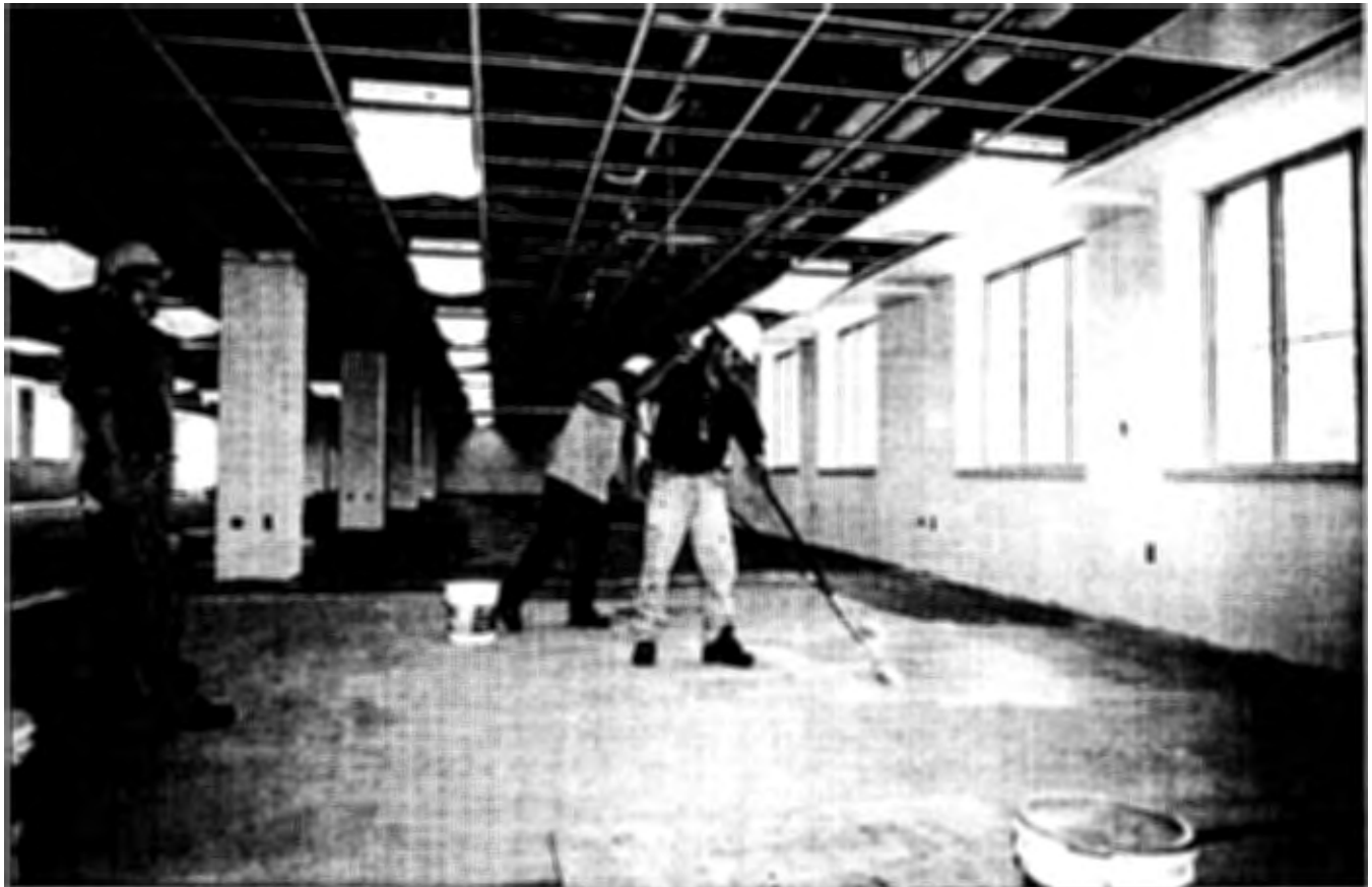
Carpet installers apply adhesive for new carpet tiles in a C-ring office bay in Wedge 1.
