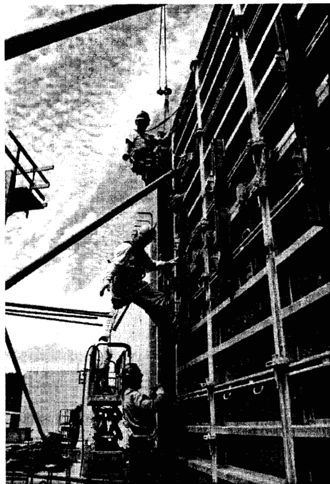
Workers secure a reinforced wall of the Remote Delivery Facility.
