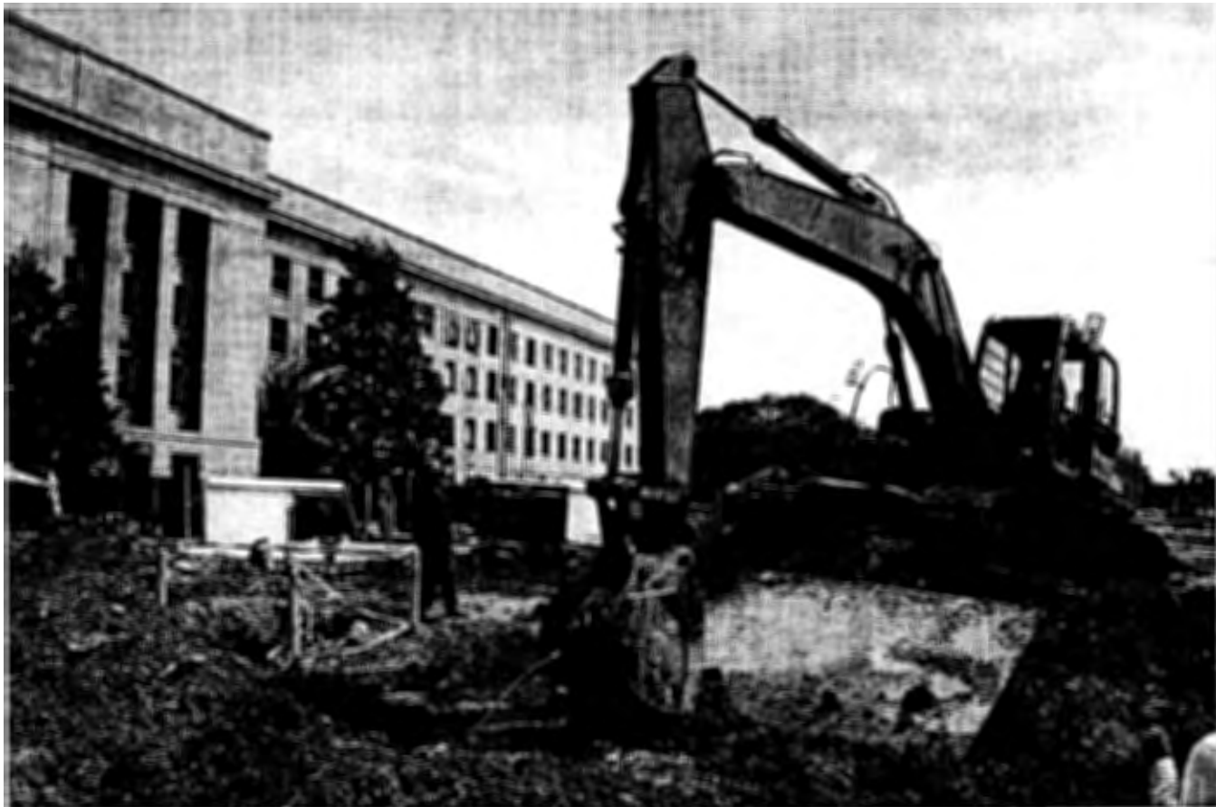
Excavation near Wedge 1 clears a trench for new telecommunication conduits.
