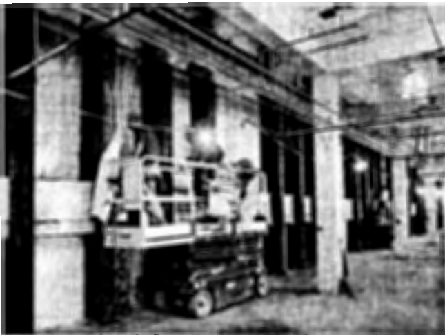
The walls of the 5th floor E-ring are reinforced with steel to improve their blast resistance capability.
