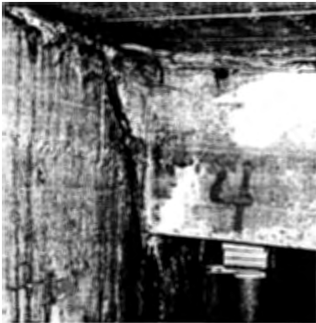
Before renovation, a person's entire hand and arm could fit through this crack in a concrete beam below the North Parking pedestrian ramp. The bridge has now been completely repaired.
