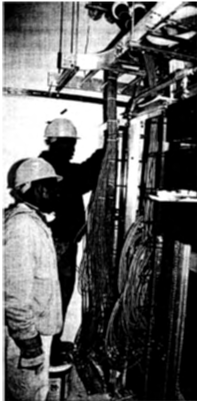
Telecommunications technicians install new telephone lines in Wedge 1.
