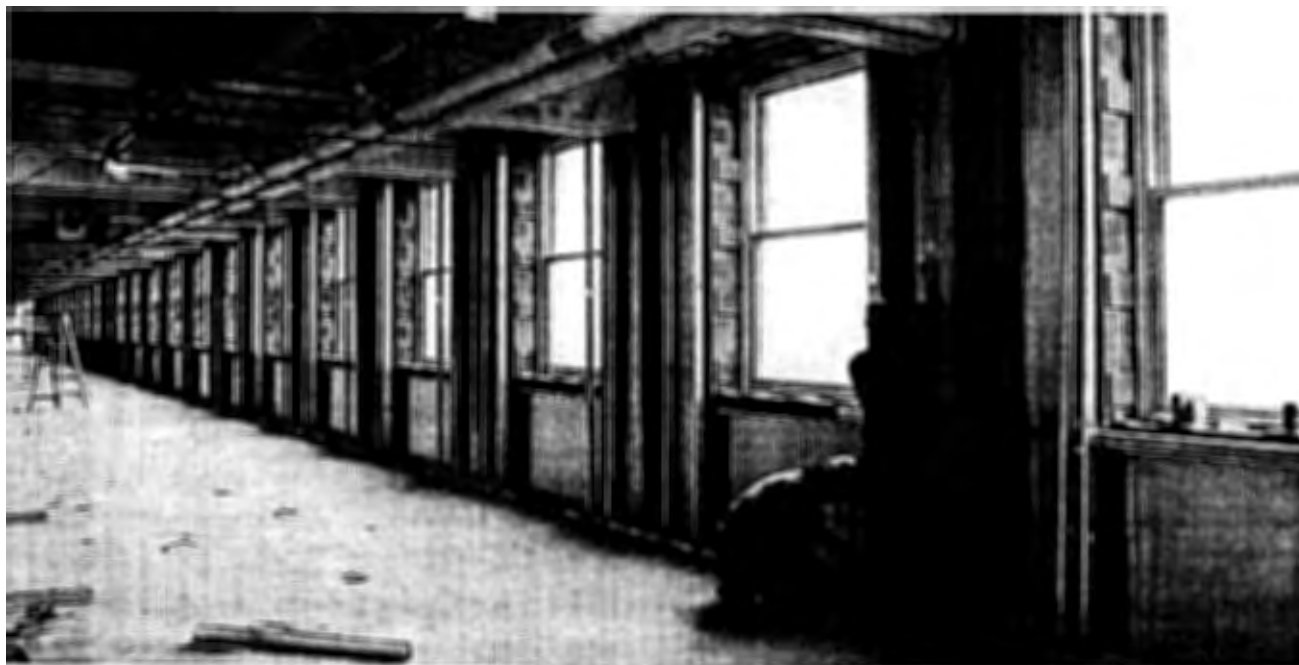
All of the Pentagon's 7,748 windows will be replaced in conjunction with the wedge-by-wedge renovation of the Pentagon. The blast-resistant windows on the E-Ring in Wedge 1 are pictured above.
