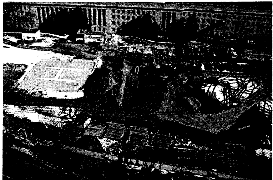
Excavation for new chilled water lines near the Pentagon Heliport.
