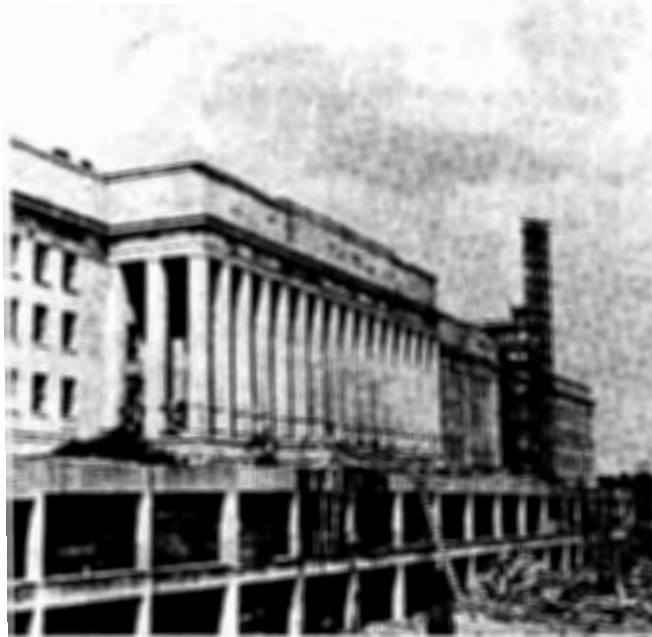
The original construction of the Pentagon took only 16 months to complete. The 29-acre structure is supported by 41,492 concrete columns.
