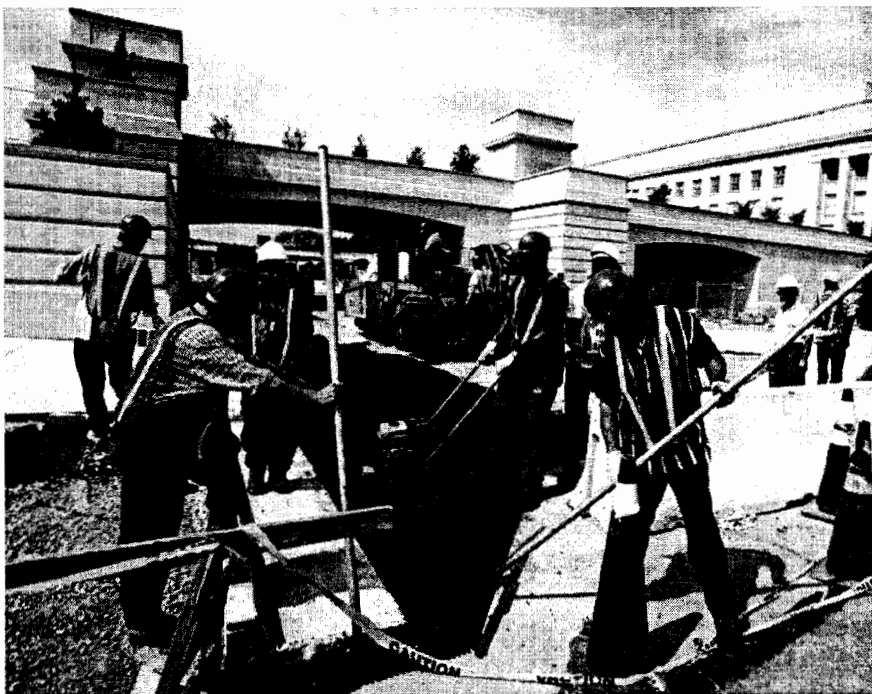
Workers pave the roadway that runs under the new South Terrace Pedestrian Bridges.
