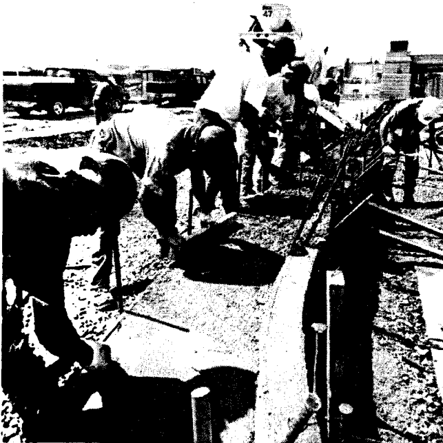
Concrete is placed and finished along a new "kiss-and-drop" area near the South Terrace Pedestrian Bridge at Corridor 2.
