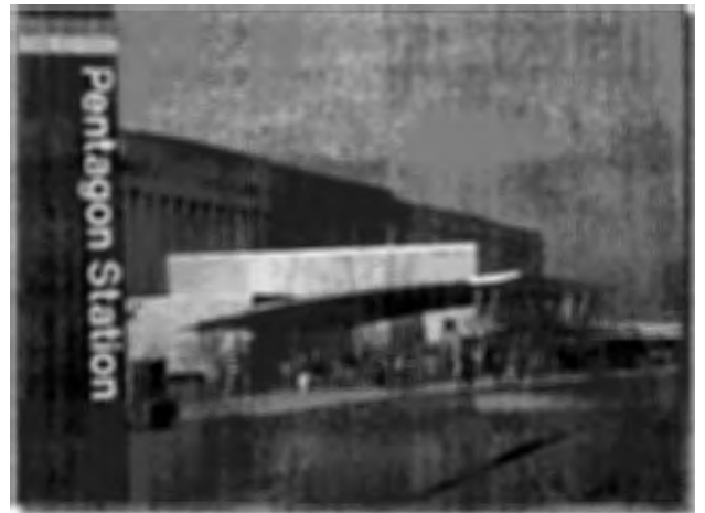
The Metro Entrance Facility (MEF) features an energy efficient roof. In December 2002, the MEF became PENREN's first LEED™ certified renovation project.
