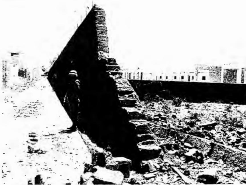
**Exterior prison compound CMU block wall with concertina wire on top. Over 1000 meters of this wall have been removed by looters in the previous weeks.**
