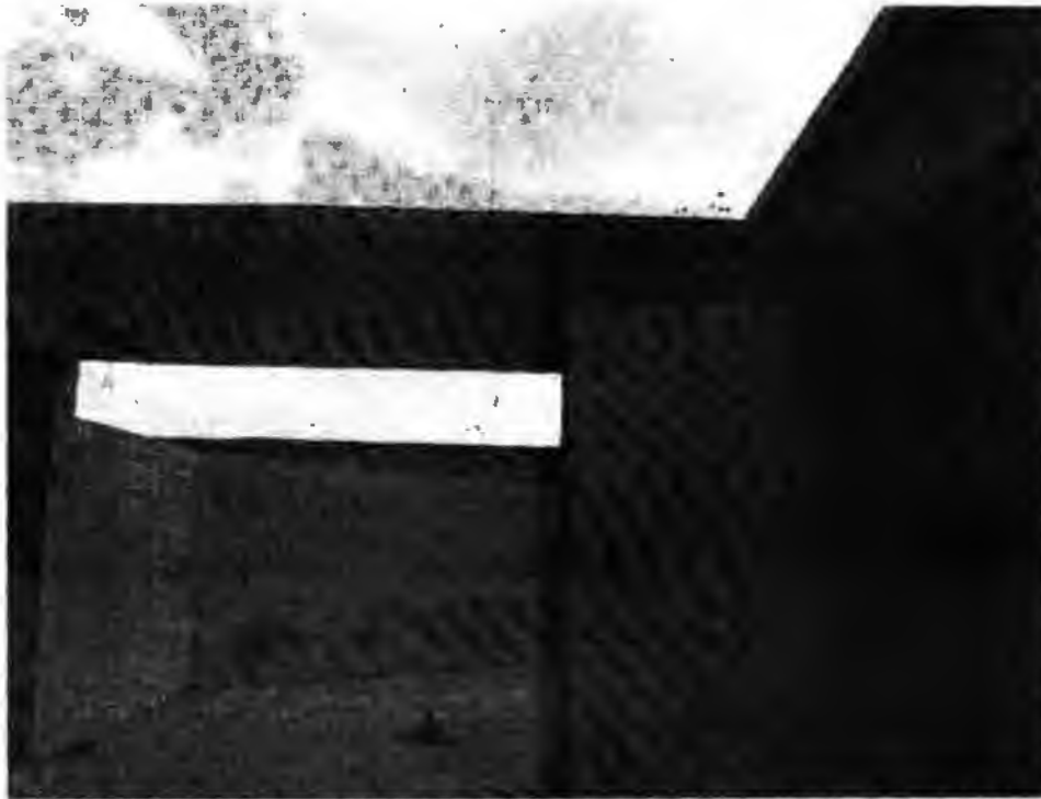
Figure 7. Breezeway roof. Typical construction (no isolation joints) at each Mosque in the compounds. Note the spalling from the breezeway and the mosque wall.
