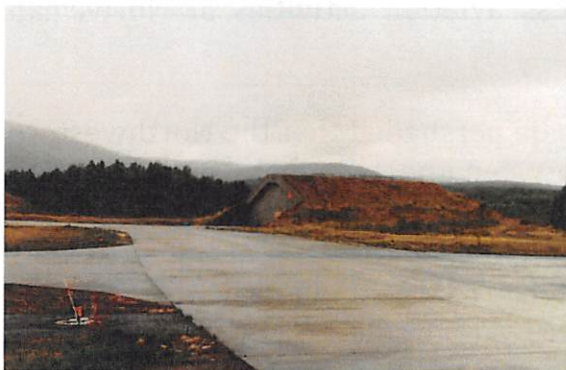
Figure 50: Not only did the Norwegians build aircraft shelters into the mountains, but they also constructed shelters for alert aircraft to both insure protection for the aircraft and their availability at a moments notice.
