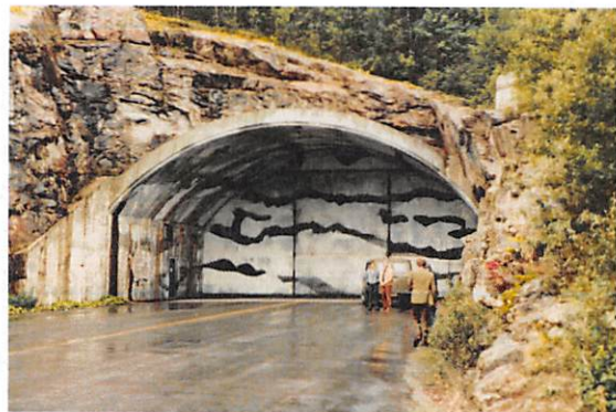
Figure 49: The entrance to this under-mountain shelter area begins with the tunnel parallel to the external “cover” then turns left into the depth of the mountain so as to insure that a direct strike at the entrance does not impact negatively upon interior operations.
