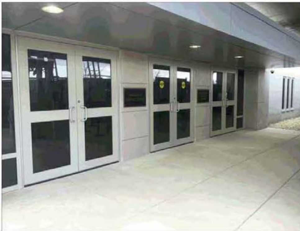
Figure 2. Entry doors to Pentagon Visitor Entrance
