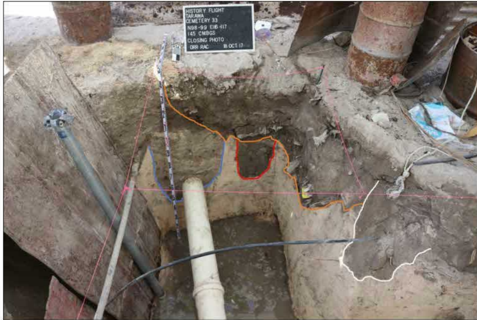
Figure 13. Excavation unit showing various soil disturbances often encountered on Betio Island. Blue line defines salt water wastewater pipe intrusion. Red line indicates disturbance for old buried electrical line (removed). Orange line shows contour of trash pit. White line indicates fresh water line placement.
